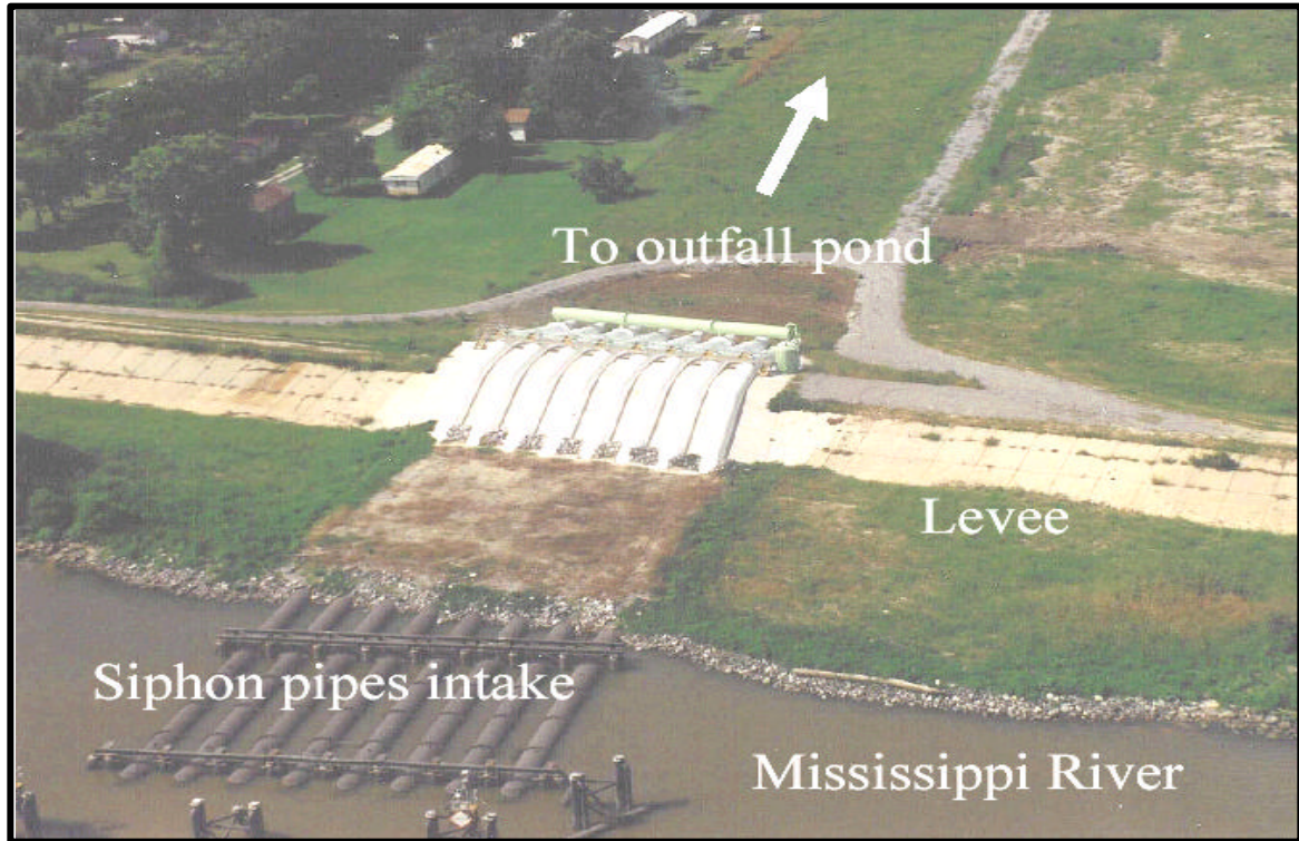
Figure 1.3: West Point a La Hache Siphon
