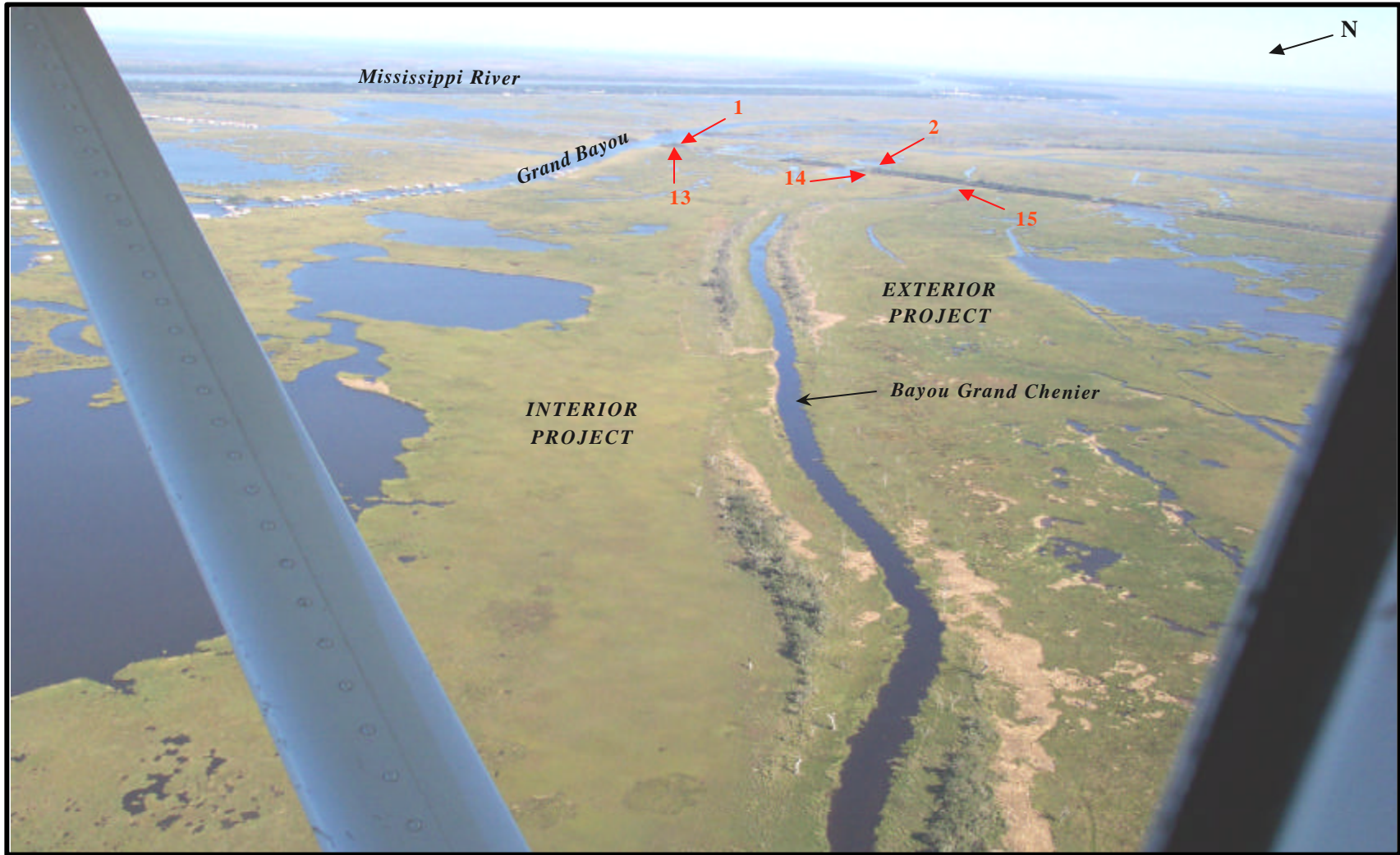
Figure 2.7: Low Altitude Photography of Bayou Grand Chenier Showing Points 1,2,13,14, and 15.
