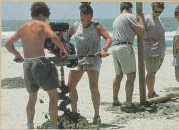
Workers constructing a dune-building fence at Racoon Island, Louisiana.
