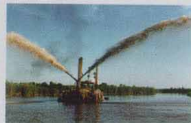
Restoring marshes with dredged sediments using a jet spray.
