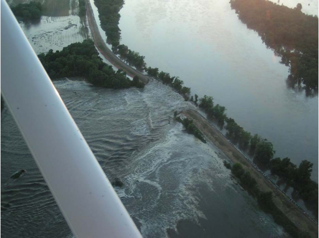
Figure 39: Levee breached before overtopping
