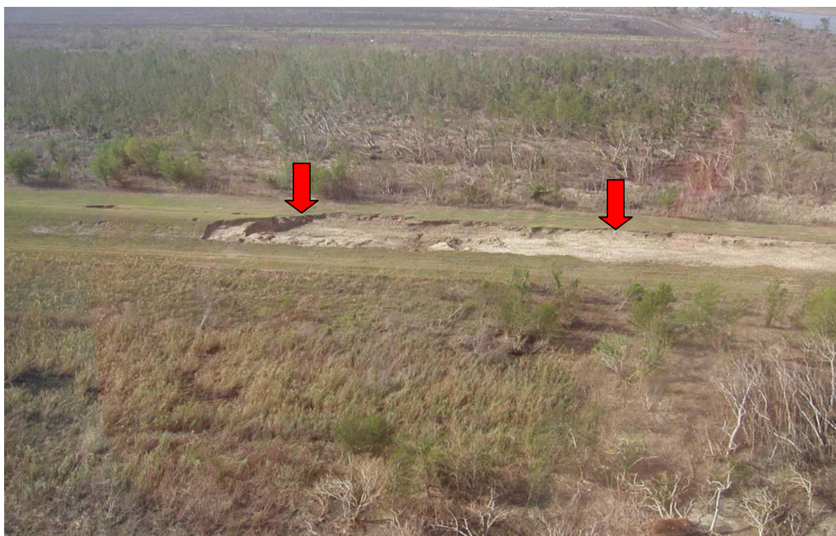
Figure B-16. High resolution pictograph of Reach 2 EBSBs showing wave erosion features (photograph provided by Dr. Paul Kemp).
