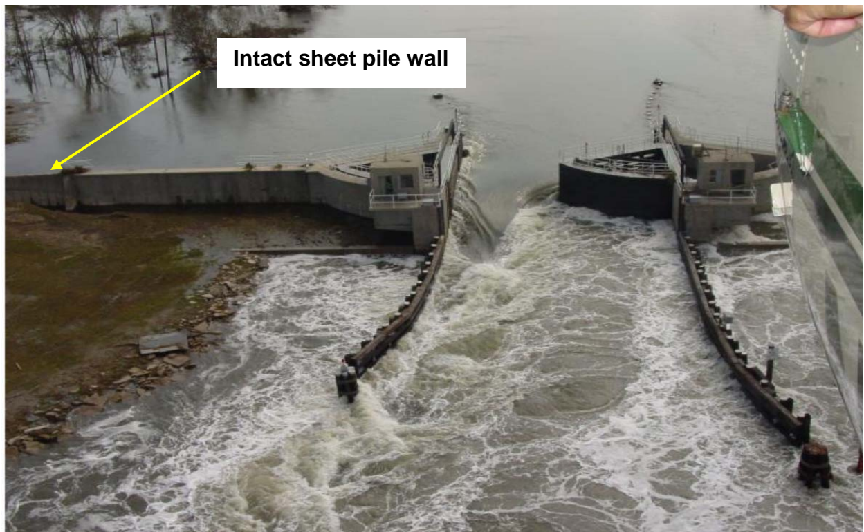
Figure 5: Photograph of Bayou Dupre navigation – water control structure taken the morning following Hurricane Katrina (EPA photograph). Photograph shows that the concrete sheet piling adjacent to the abutment of the structure are intact.
