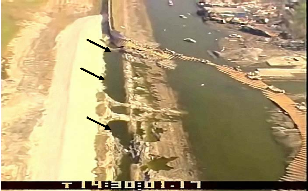
Figure 46: Video frame from aerial survey of Lower 9 th Ward on September 14, 2005 – South Breach (USACE Video Survey). Light ground area to left is breach repair.
