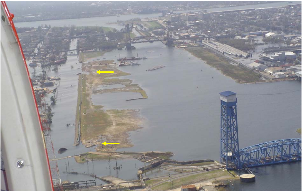
Figure 47: Aerial photograph showing ‘depressions’ outside the Lower 9 th Ward floodwall before breach repair operations were initiated (USACE photograph).
