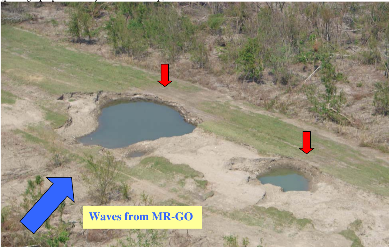
Figure B-17b. Aerial photograph of Reach 2 EBSB showing wave erosion features (photograph provided by Mr. Less Harder).
