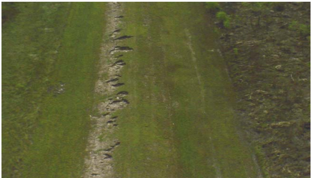
Figure 23: Wave erosion of floodside of EBSBs. Note wave eroded ‘mowed strip’ on flood side.
