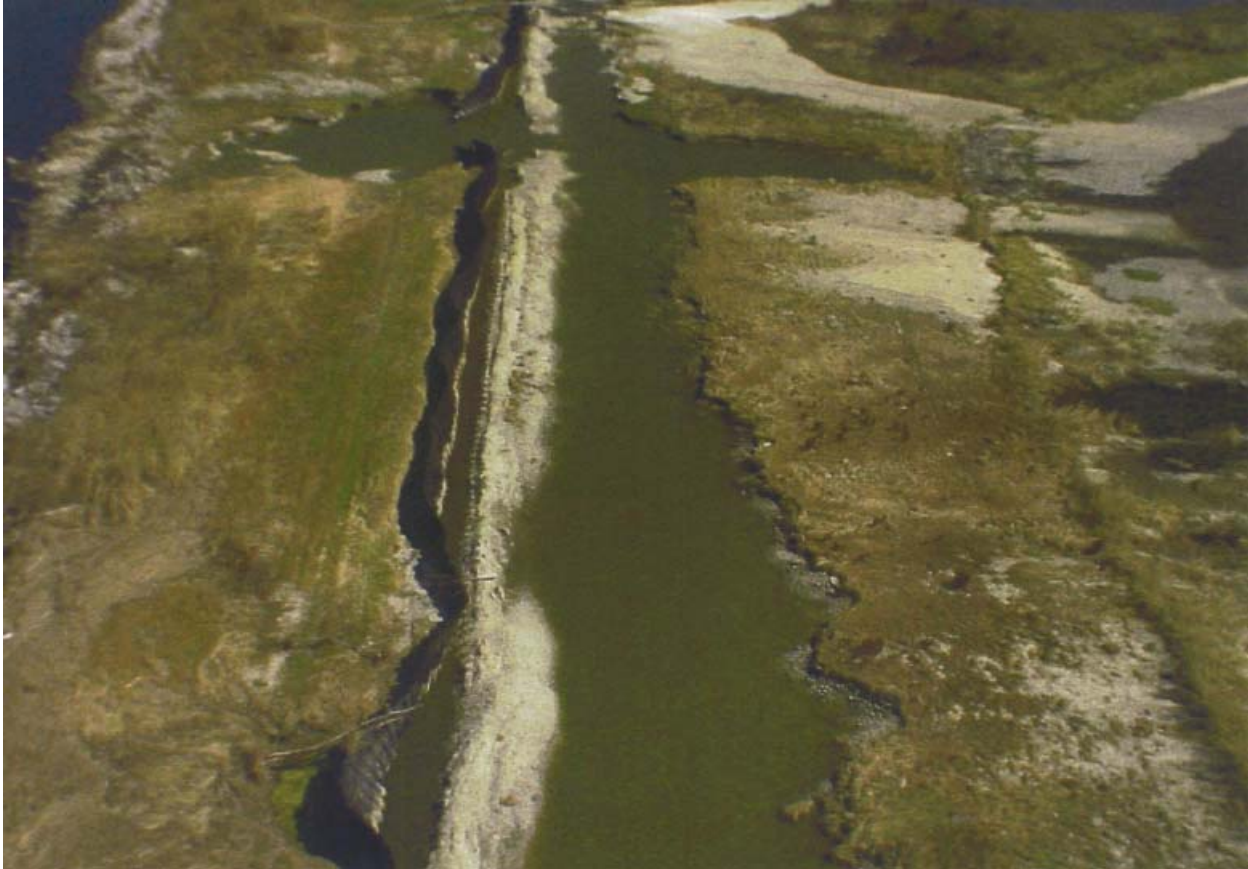
Figure 26: Sheet piling overtopping erosion of EBSBs.
