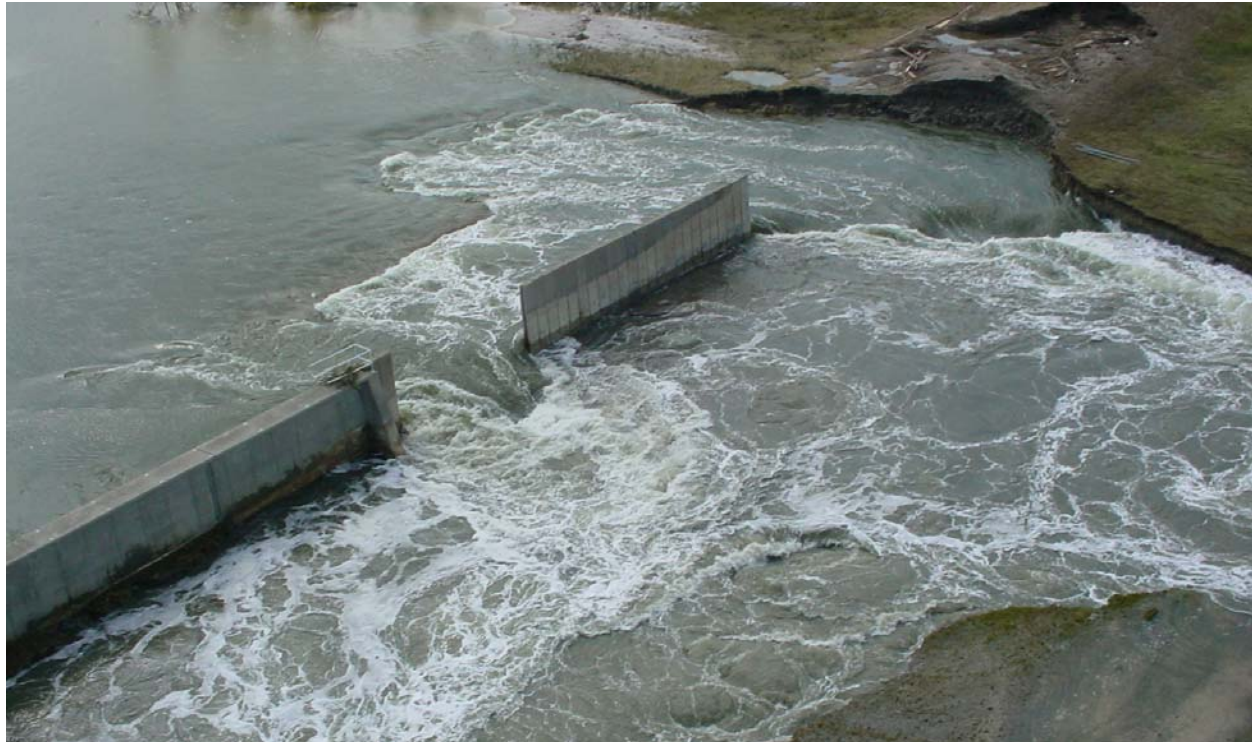
Figure 7: Aerial photograph of Bayou Dupre north side breach developing during ebb tidal flow following Hurricane Katrina (USACE photograph). Note breach development at EBSB – concrete sheet pile interface.
