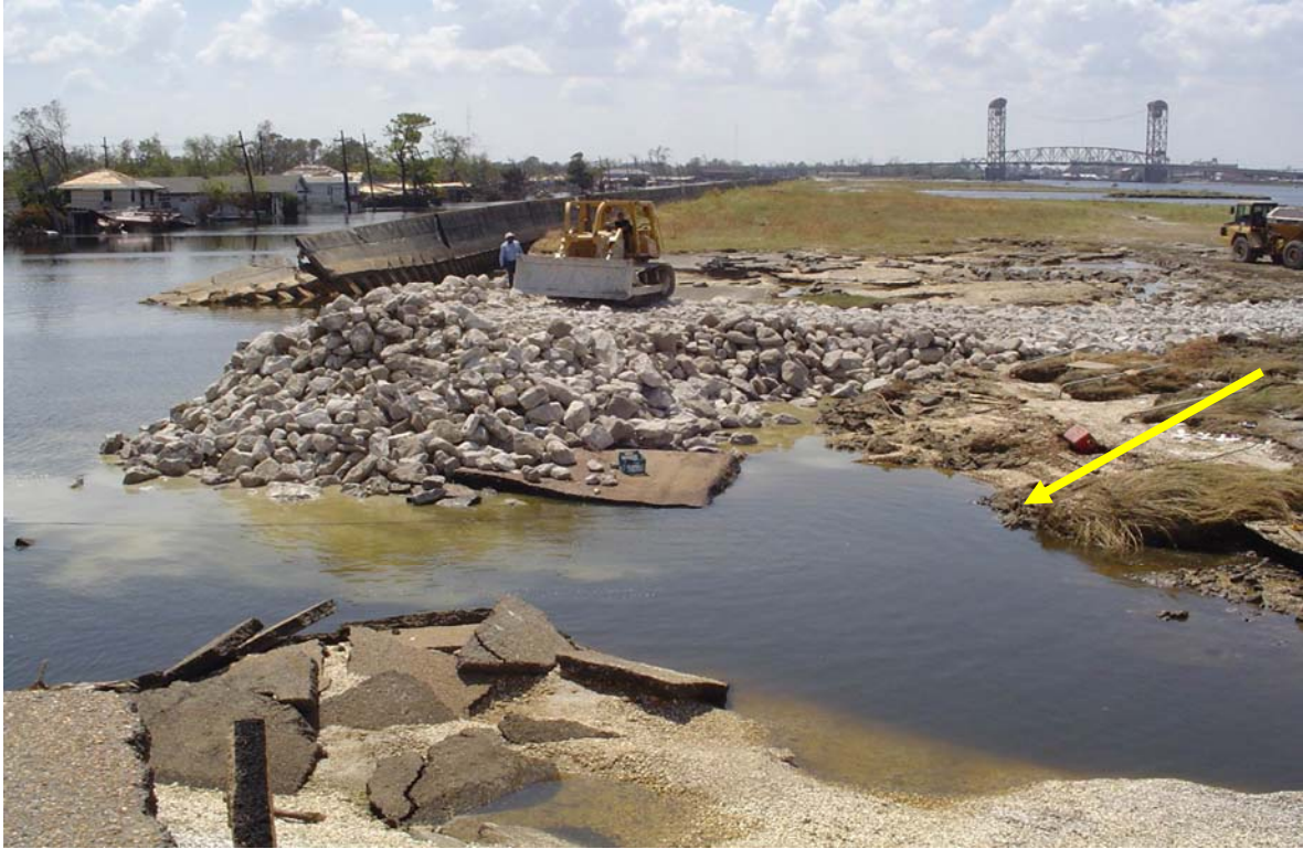
Figure 49b: North Breach during initial repair period before hole outside of the floodwall is covered (USACE photograph).
