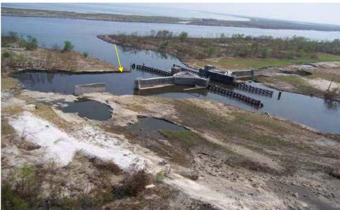
Figure 51. Bayou Dupre Control Structure
