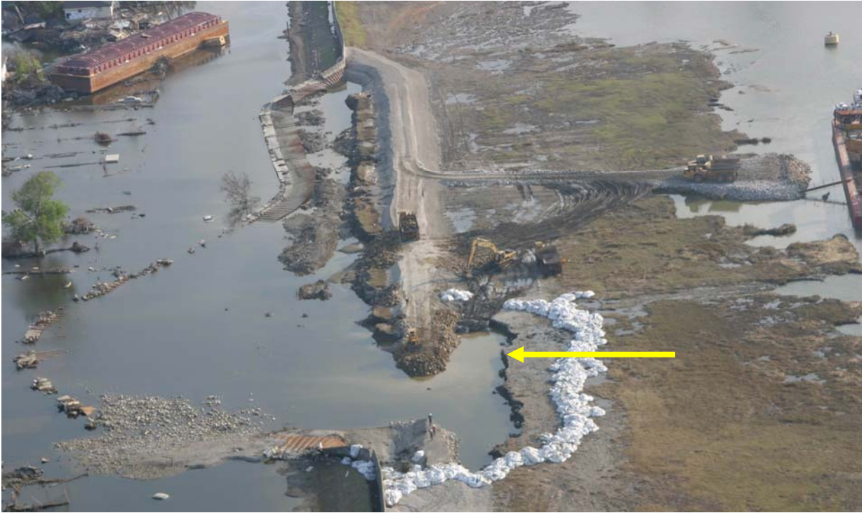
Figure 48: South Breach during initial repair period before hole outside of the floodwall is covered (USACE photograph).
