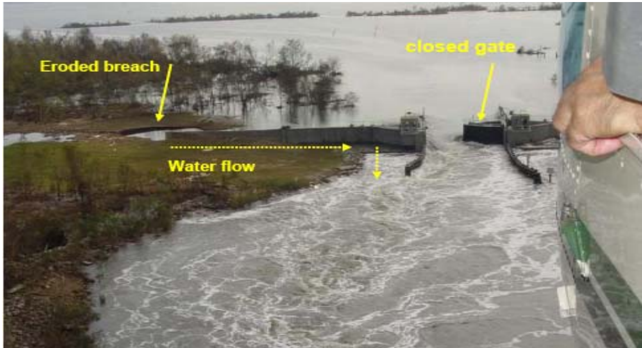
Figure 10: Large eroded breach at the contact between the north end of the concrete navigation lock structure at Bayou Dupre and the adjacent EBSB (EPA 2005).
