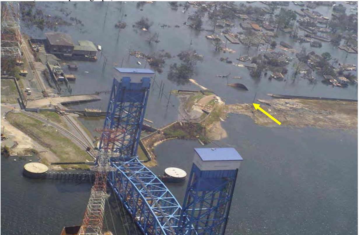
Figure 49a: North Breach during initial repair period before hole outside of the floodwall is covered (USACE photograph).
