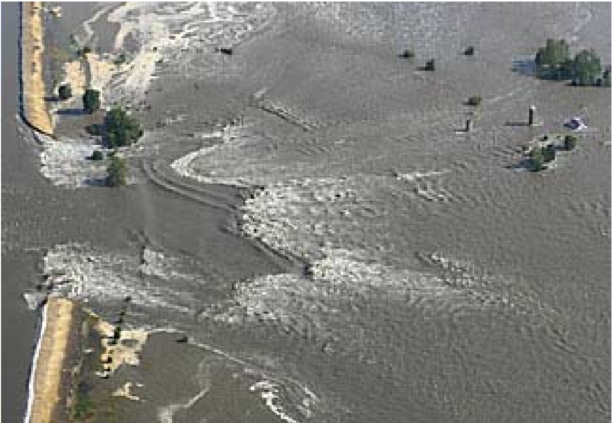
Figure 41: Levee adjacent to windmill developed breach prior to overtopping
