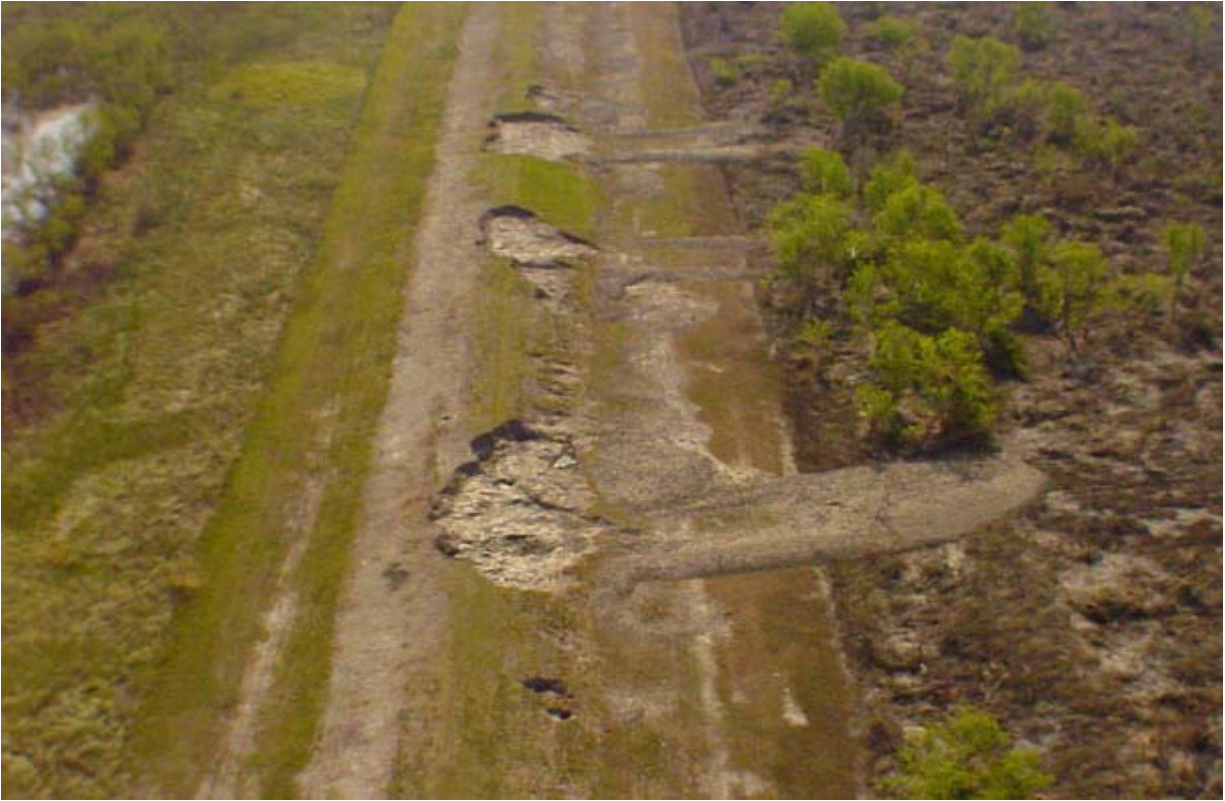
Figure 24: Overtopping erosion of protected side of EBSBs.
