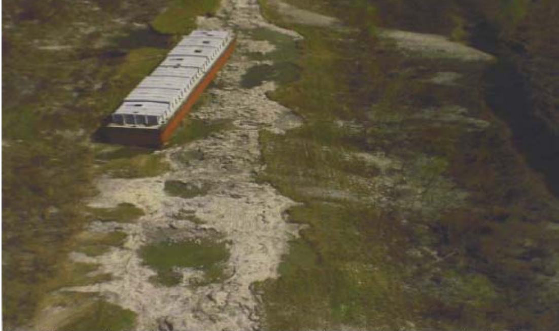
Figure A4. Severely degraded levee. Evidence of overtopping indicated by overwash sediment deposits on back side. Channel present just to south (top edge) of the barge. Backside elongated sediment deposit suggests high overflow. Traces of deposited sediment at front of the channel mouth also suggest outflowing water. Channel likely formed on outflow. Lowest spots on the degraded levee likely served as outflow channels for water exiting the polder following storm's passage. Situation in lower half of photo is less clear.
