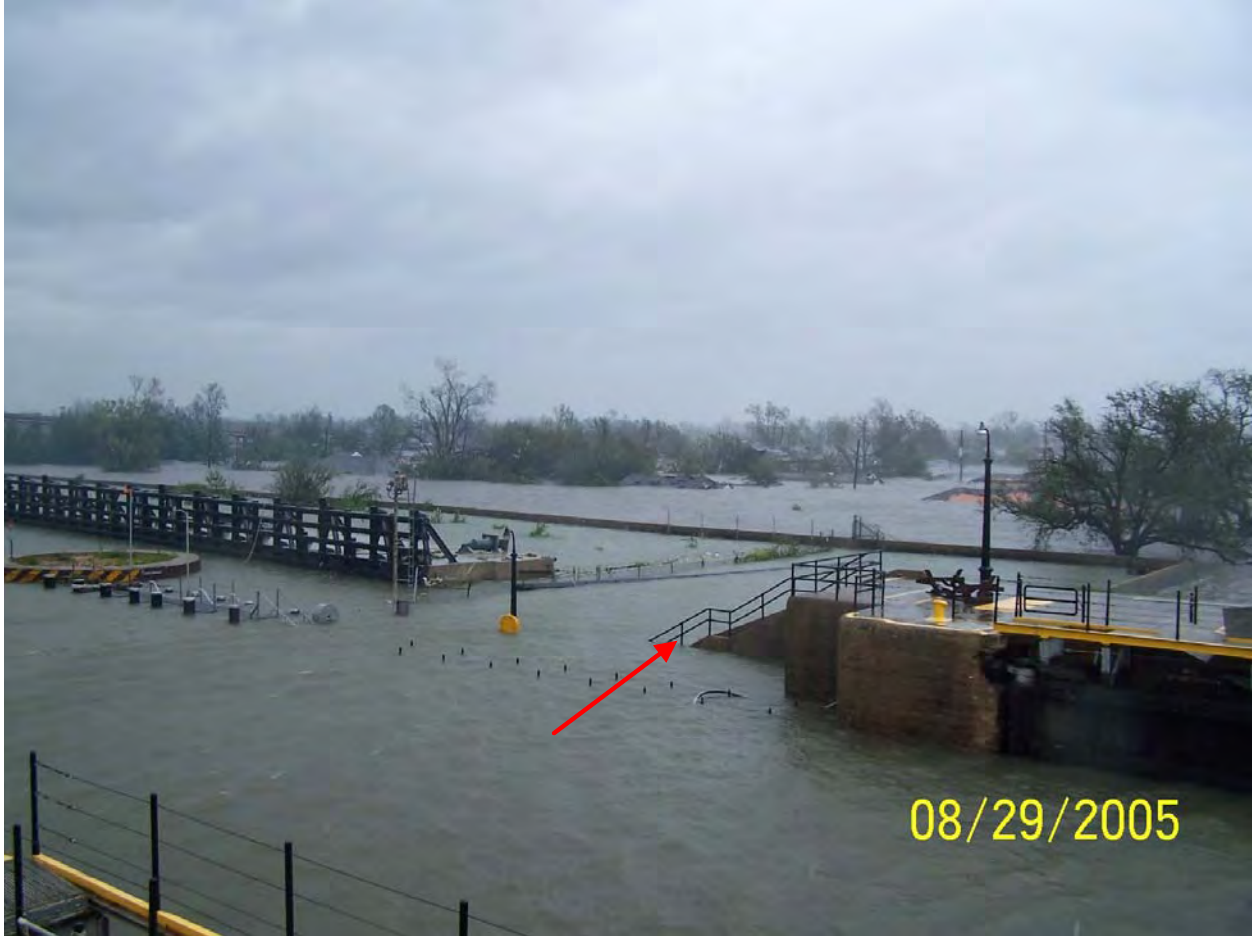
Figure 1-60. Time 11:47, picture 100_0502. Red arrow shows location surveyed. Looking east-northeast into Lower Ninth Ward.
