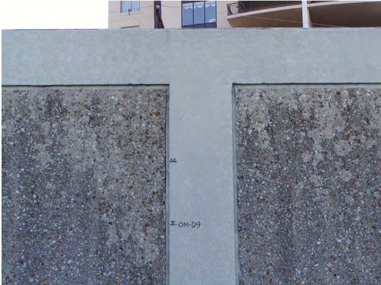
Figure 1-30. Time 11:00 on 8/29/05, elevation 12.5 ft (top of floodwall), 10.2 ft (peak of 2 ft waves), 9.2 ft (average water level at OM-09)
