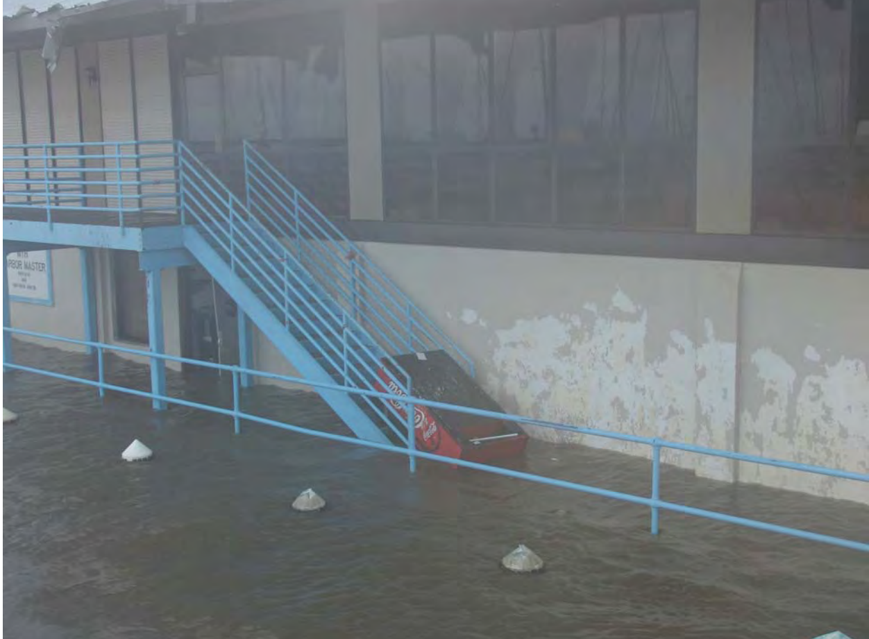
Figure 1-18. Picture DSC02263.JPG taken at 1538:54 (CDT) on 8/29/05, elevation 6.5 ft. Looking southeast. From left to right, water level is 0.5, 0.7, 0.7, and 0.9 ft below the center of the lower rail.
