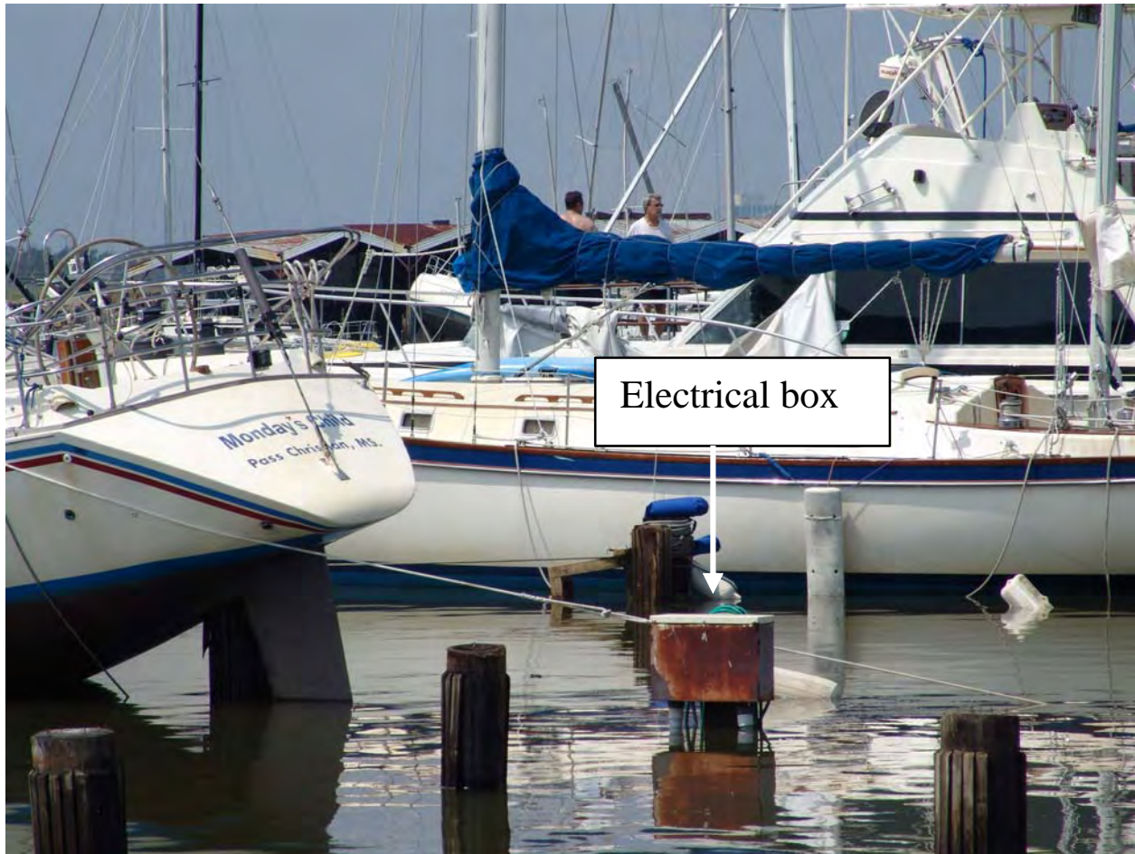
Figure 1-25. Picture DSC02338.JPG taken at 1132 (CDT) on 8/30/05 elevation 4.4 ft. Electrical box at east end of third row of docks
