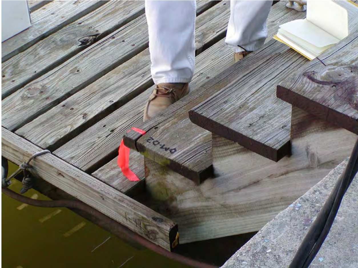
Figure 1-27. Time 1:30 on 8/29/05, elevation 3.7 ft. Top of first step on finger dock
