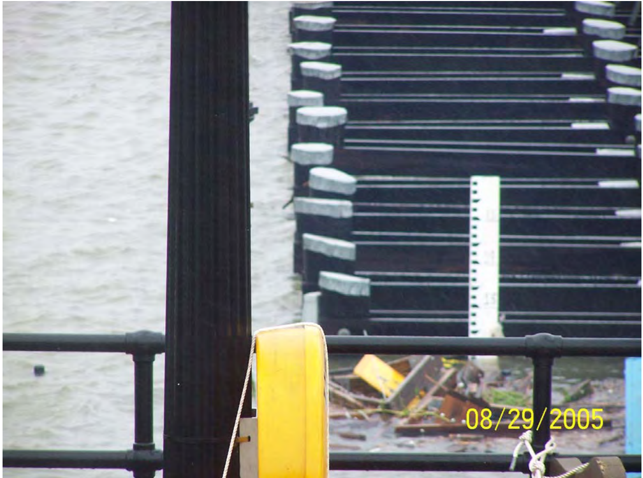
Figure 1-61. Time 11:50, picture 100_0507, looking north.
