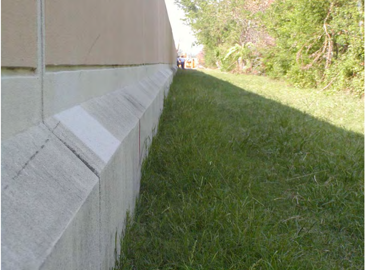
Figure 1-82. Attempt to show possibility of minor scour along west floodwall, south of 17th Street Canal breach.
