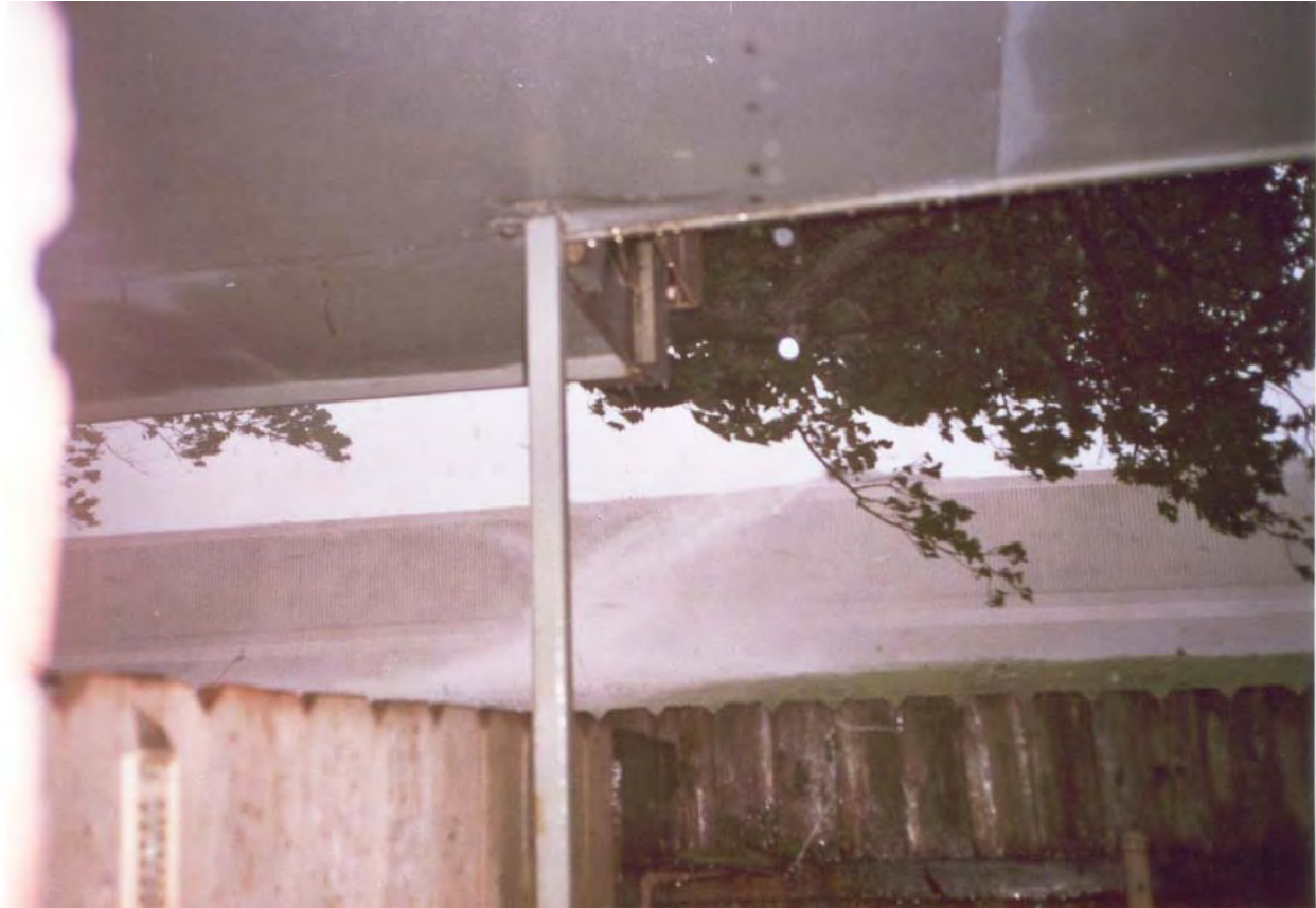
Figure 1-87. Wave spray or splash (left of tree limb) at west wall of 17th Street Canal north of Veterans Blvd and 1.0 mile south of Hammond Hwy. The individual who took this picture stated that the tree limb obscures the crest of a wave.
