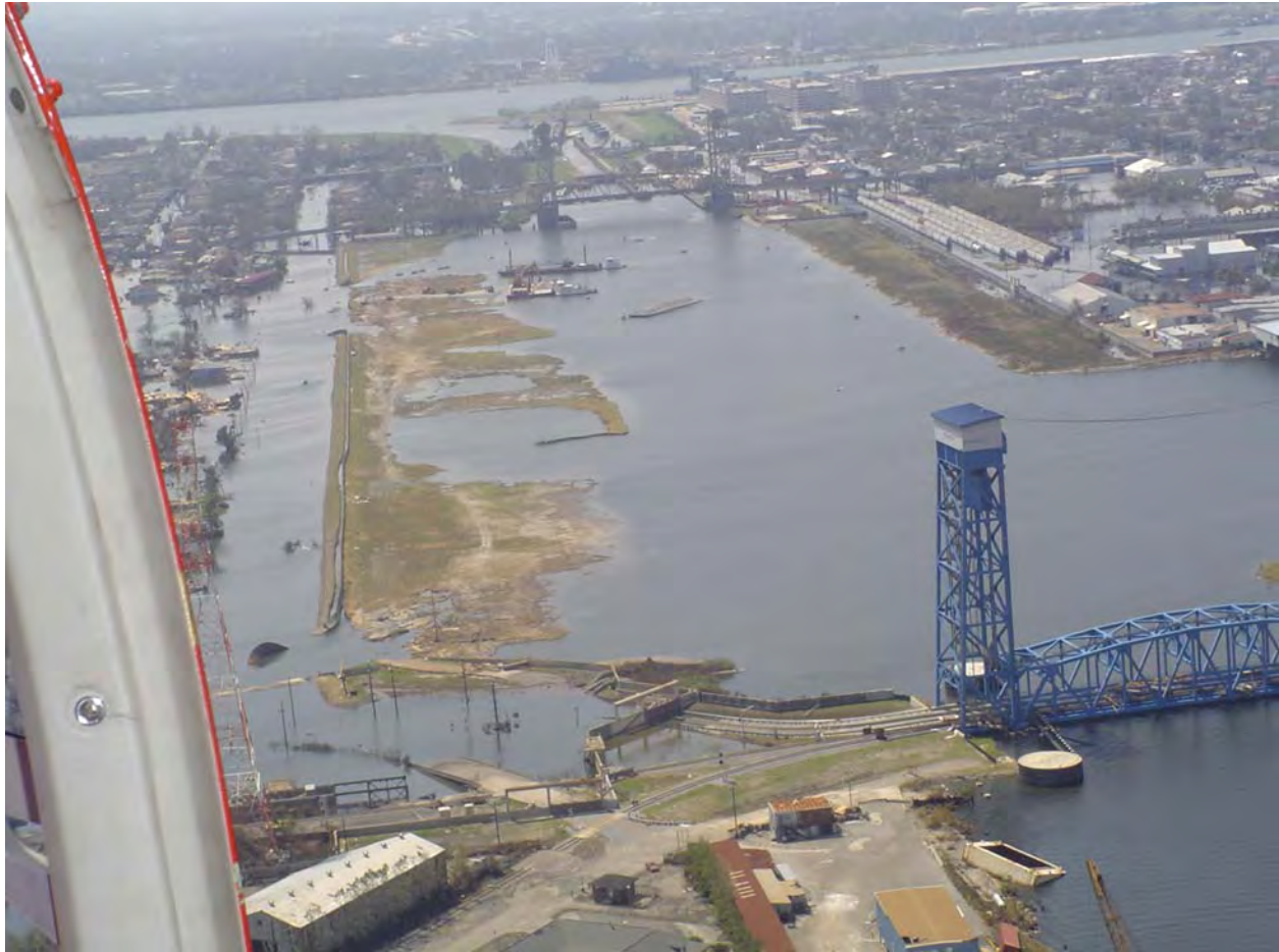
Figure 1-69. Florida Avenue railroad bridge (blue), two breaches on east side of IHNC into Lower 9 th Ward, and IHNC lock at top of picture. Picture looking south-southwest. Note debris on railroad bridge.
