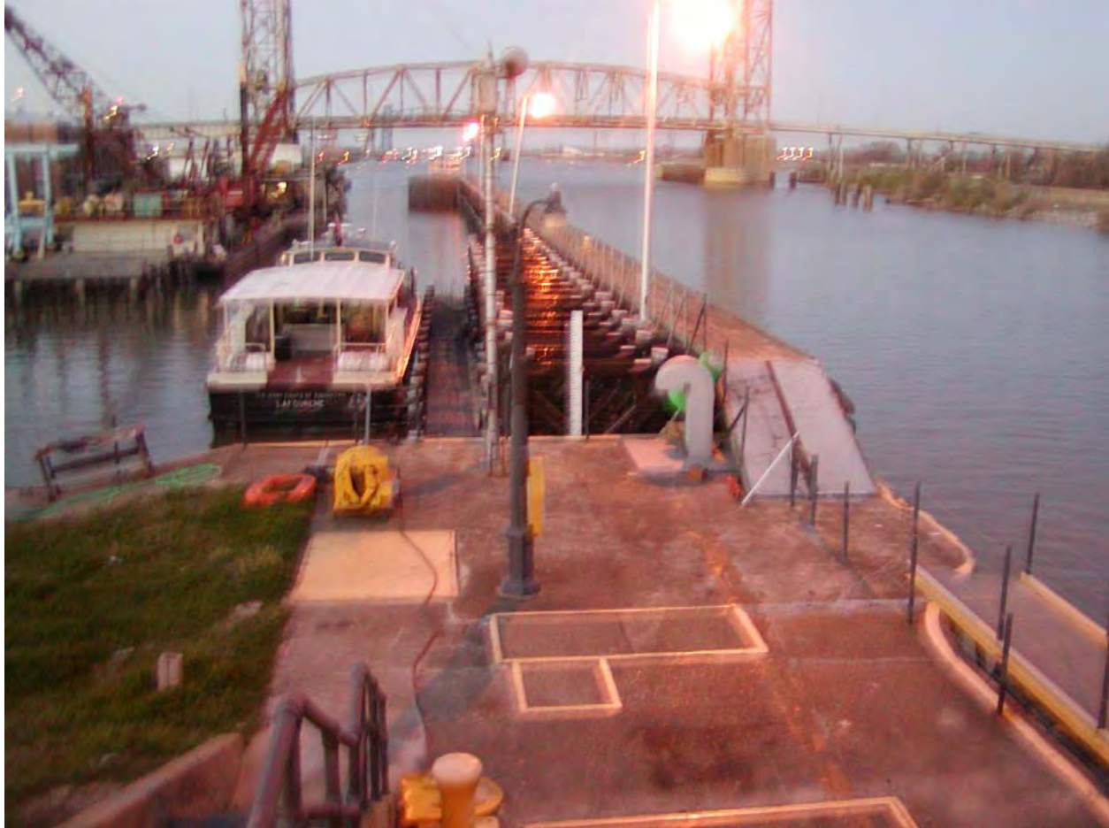
Figure 1-58. Staff gage from viewing location during storm. Picture looking north. Claiborne Avenue bridge in the background.
