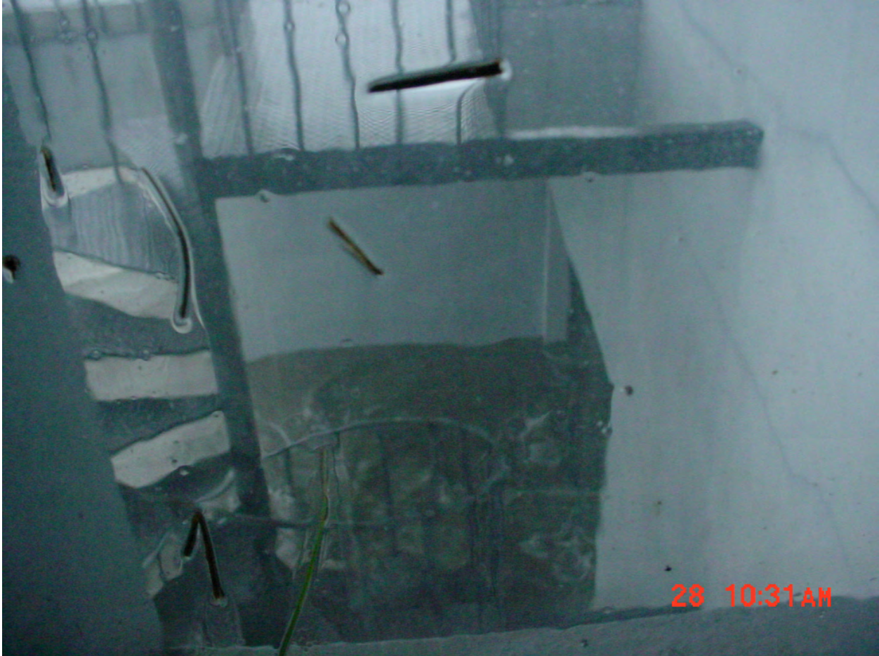
Figure 1-43. Time = 10:31 AM, APH-02. Wall north of west spiral staircase.
