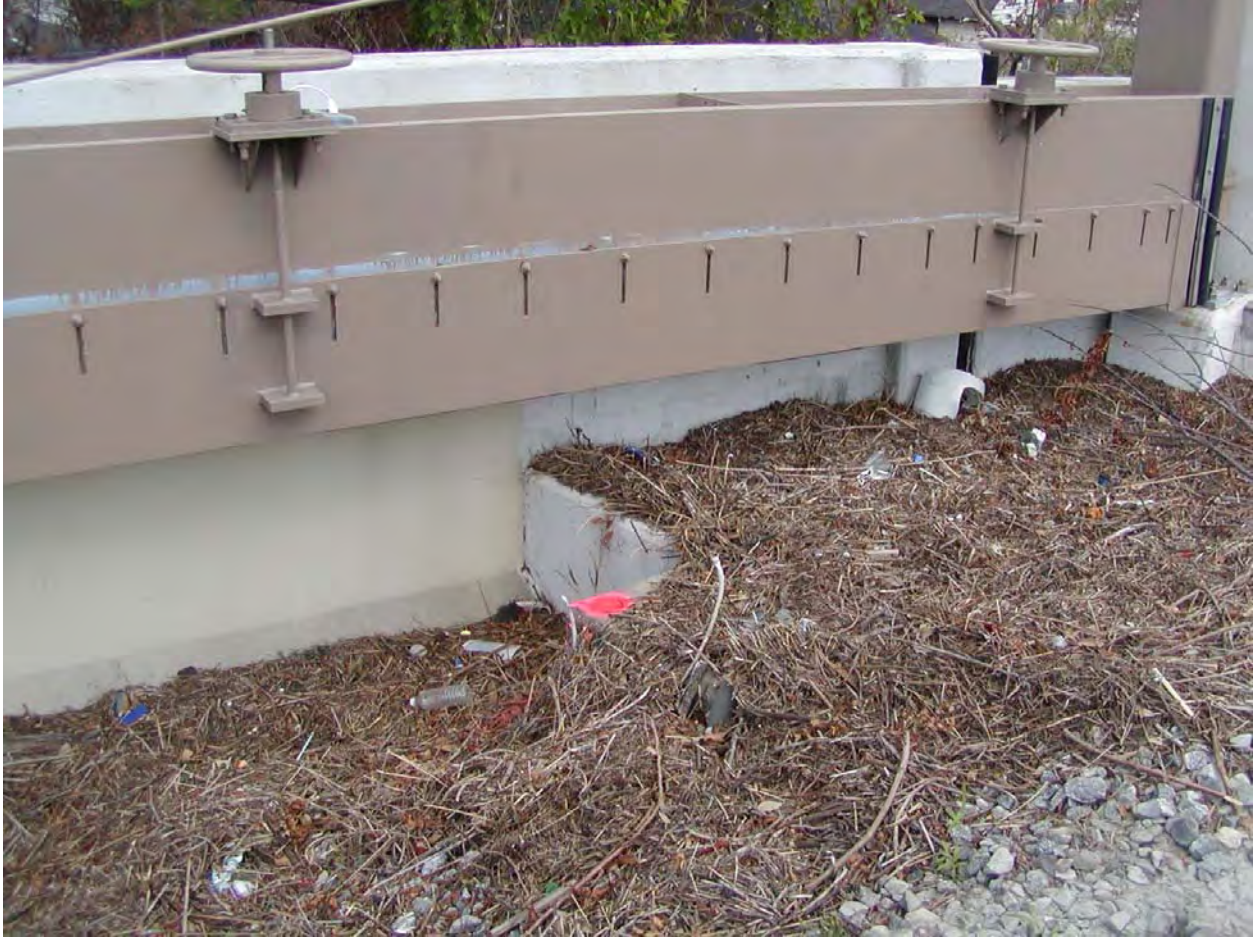
Figure 1-95. East floodgate at OP#3 at south end of London Avenue Canal. High water mark LA 1018 at top of painted concrete wall.
