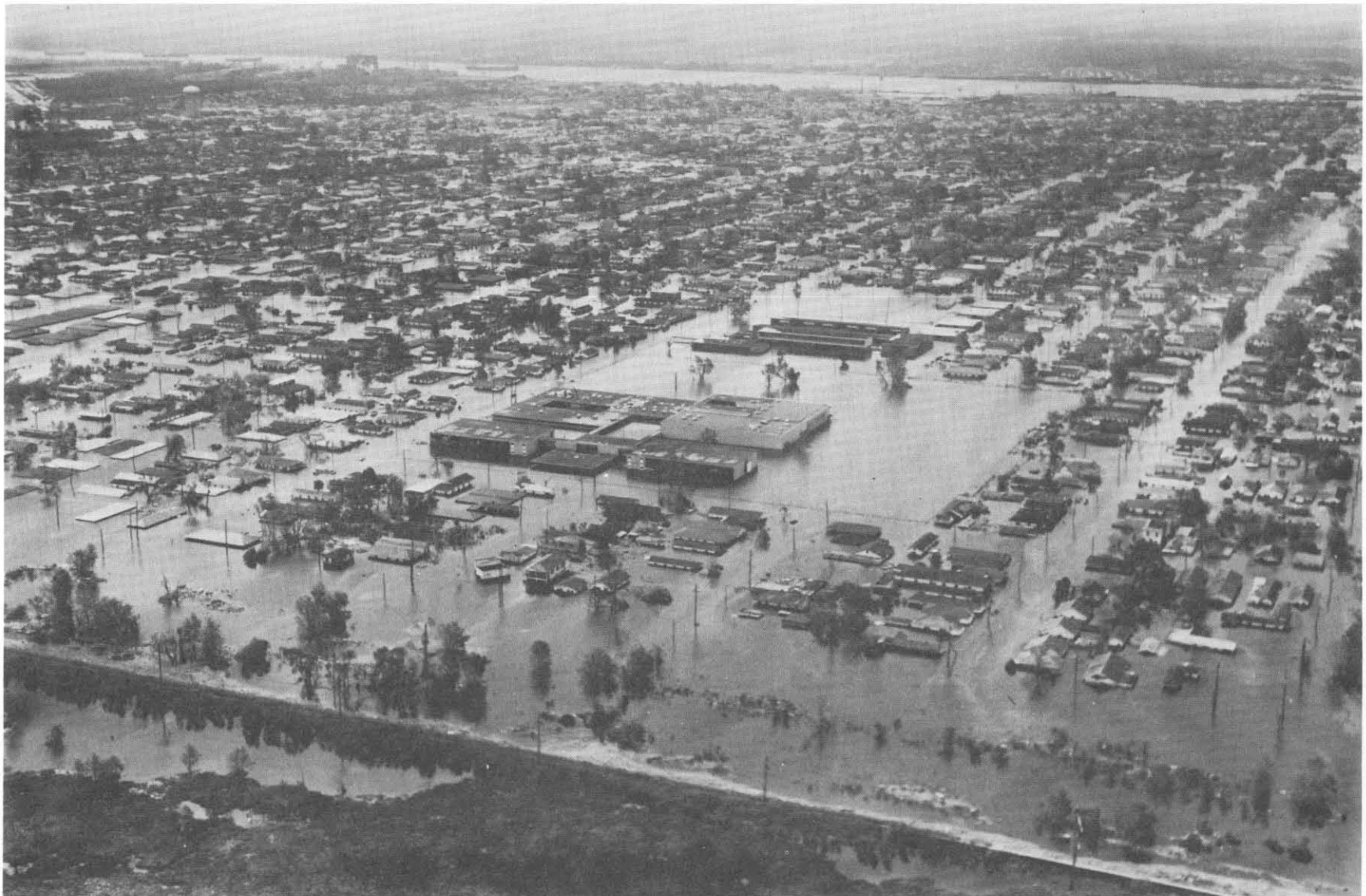
HIGH TIDE FLOODING EAST OF INNER HARBOR NAVIGATION CANAL IN ORLEANS PARISH NEW ORLEANS, LA., 11 SEPTEMBER 1965
