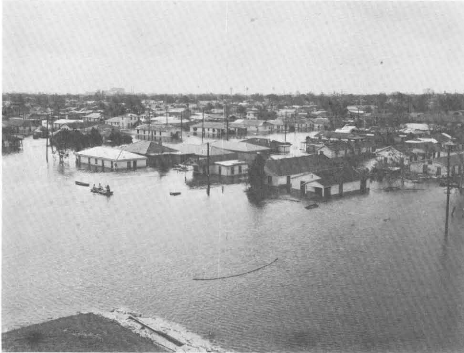
HIGH TIDE FLOODING EAST OF INNER HARBOR NAVIGATION CANAL NEW ORLEANS, LA., 11 SEPTEMBER 1965
