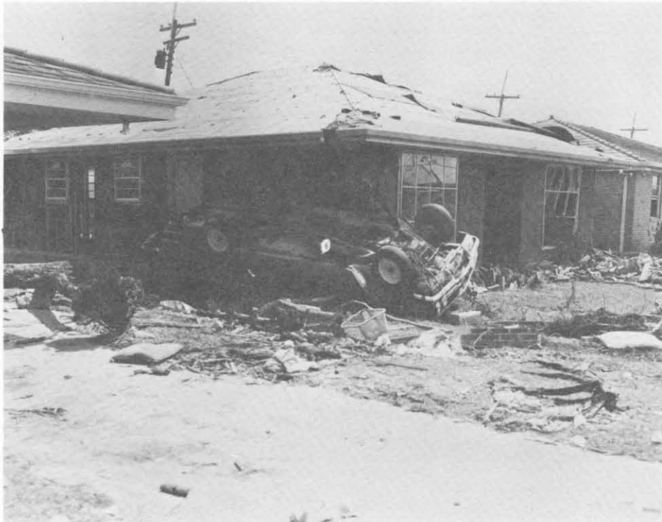
WATER AND WIND DAMAGE NEW ORLEANS, LA.
