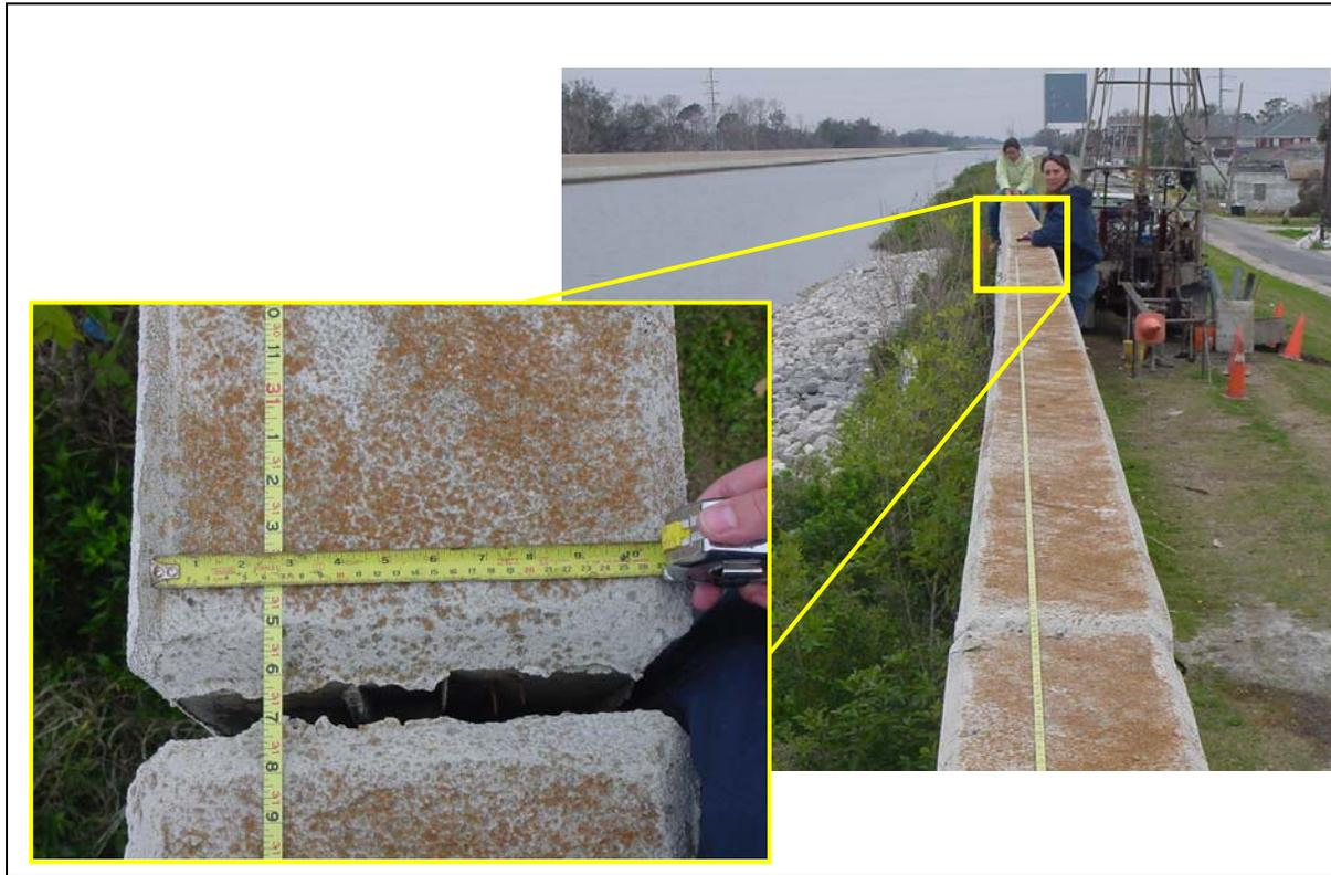
Figure 8.75: View of floodwall displacement on the west bank of the 17<sup>th</sup> Street Canal.
