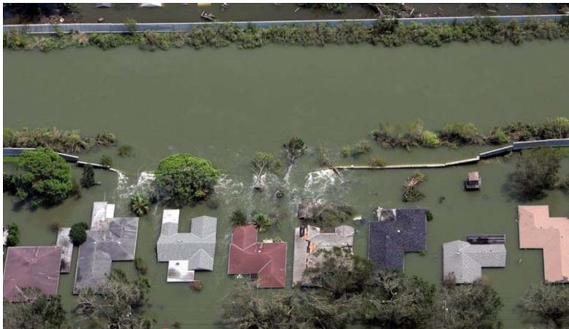
Figure 8.110: Overhead view of the breach section on the west bank near the north end of the London Avenue Canal.
