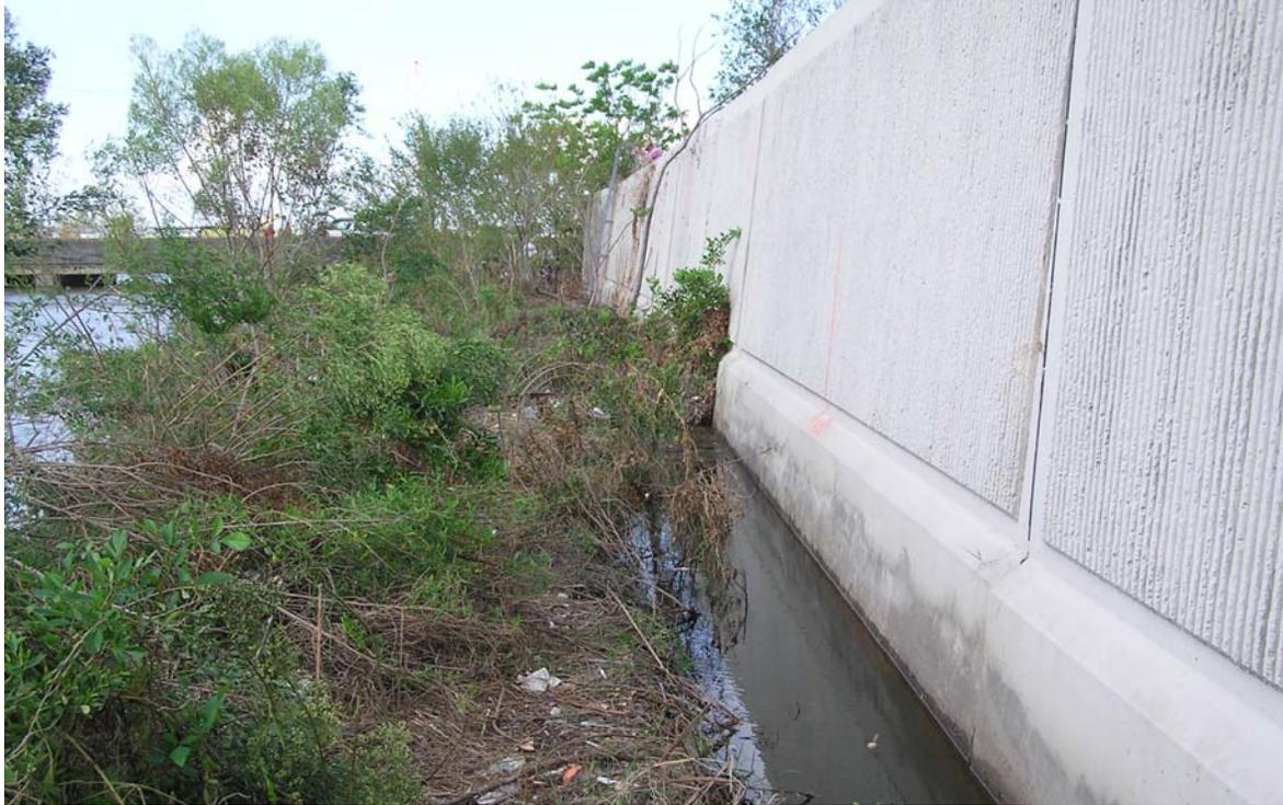
Figure 8.114: Water-filled gap at outboard side of east bank distressed section.
