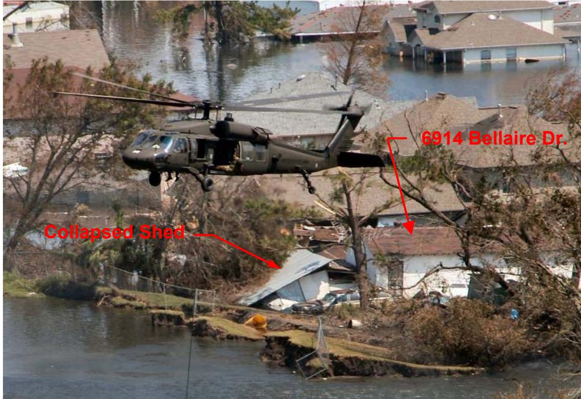
Figure 8.30: Side view of the collapsed shed pushed into the house at 6914 Bellaire Drive as illustrated in the cross-section of Figure 8.27.
