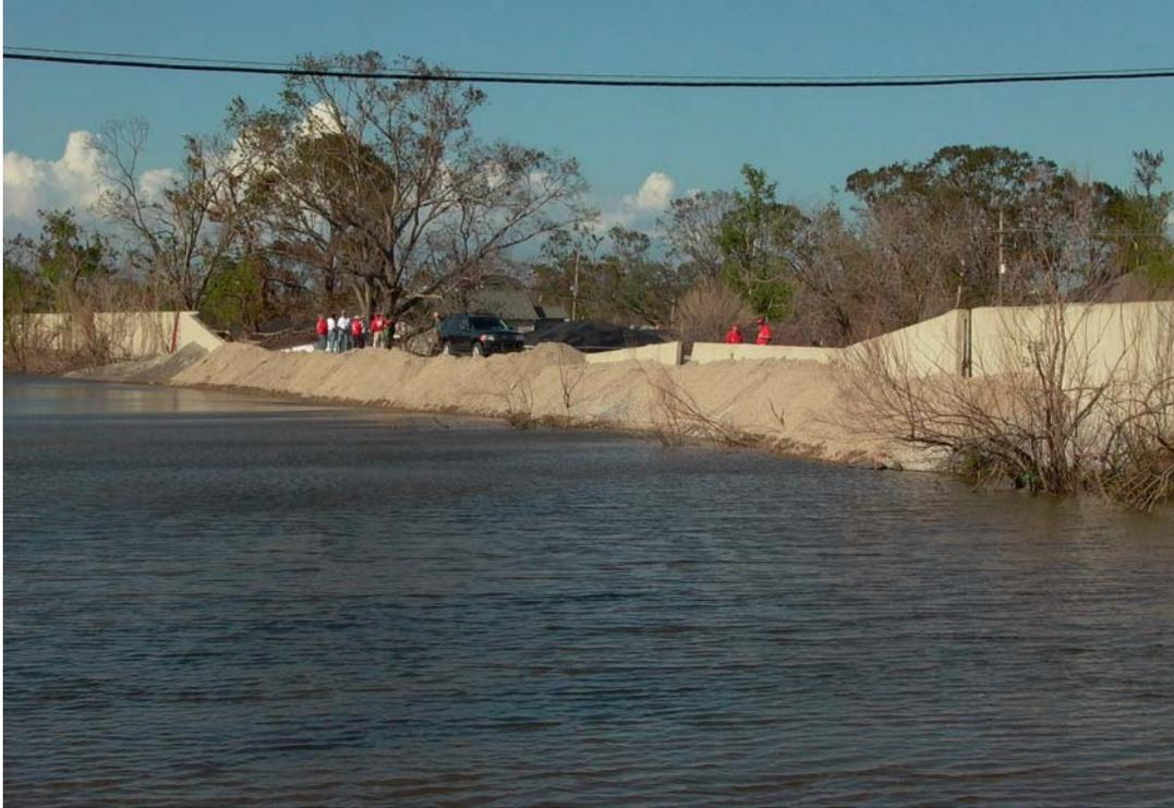
Figure 8.109: View of the breach near the south end of the London Avenue Canal from the canal side in late September of 2005.
