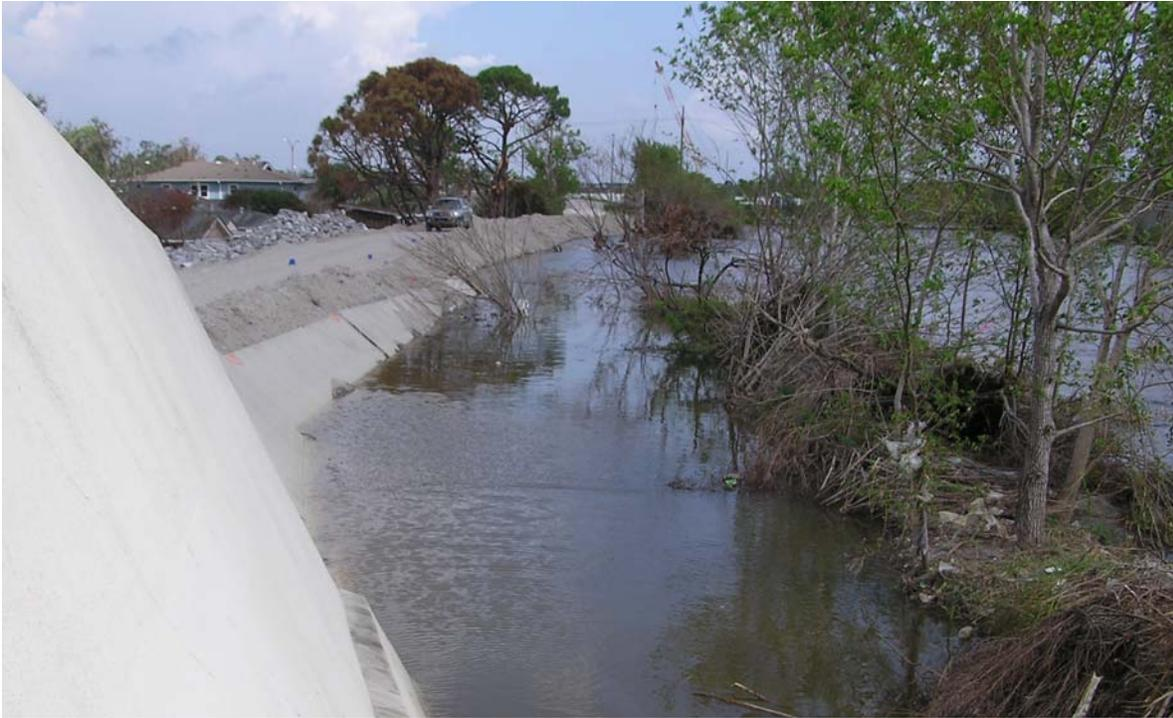
Figure 8.112: View of the west bank breach near the north end of the London Avenue Canal from the south end showing the outboard side embankment section still in place.
