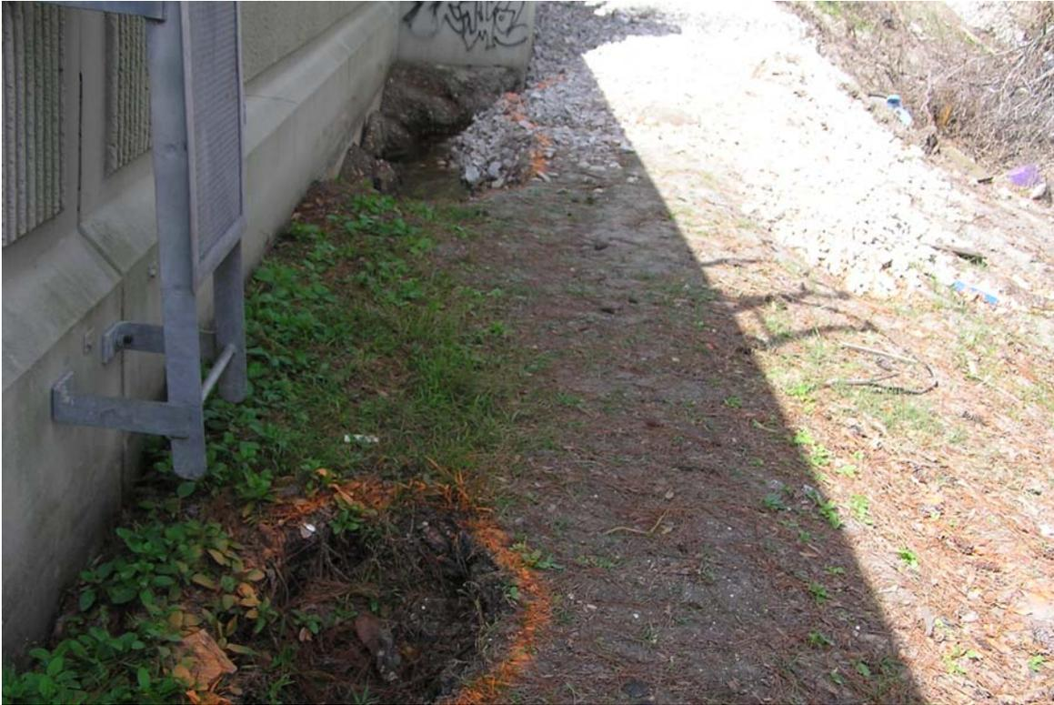
Figure 8.116: Sinkholes along the contact at the inboard side base of the floodwall and the levee crest.
