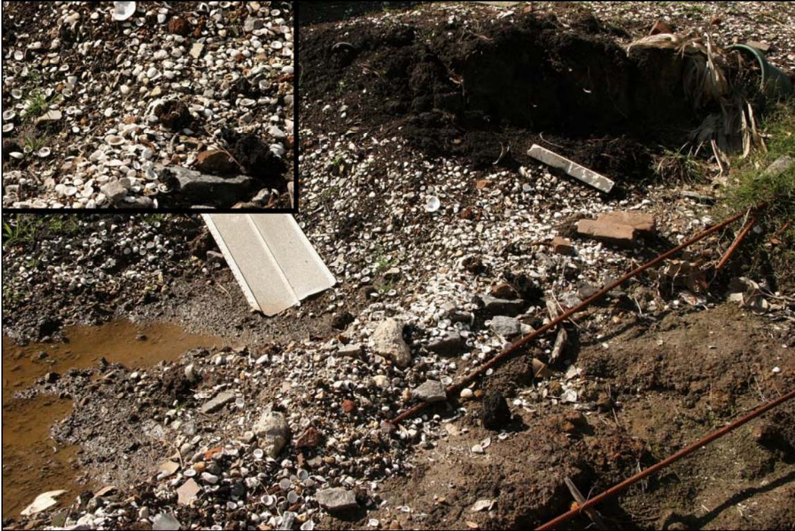
Figure 3.20: Bivalve shells ejected by high pore pressures emanating from toe thrusts on landside of failed levee at the 17 Street Canal (detail view at upper left). These came from a distinctive horizon at a depth of 2 to 5 feet below the pre-failure grade (photo by C.M. Watkins).
