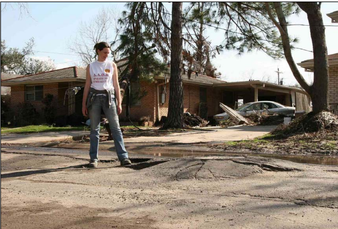
Figure 3.28: Upper photo shows gross near-surface settlement of homes in the Lakeview neighborhood, close to the 17 th Street Canal breach. Most of the homes were constructed from 1956-75 and are founded on wood piles about 30 feet deep. The lower photo shows protrusion of a brick-lined manhole on Spencer Avenue, suggestive of at least 12 inches of near surface settlement during the same interim (photos by J. D. Rogers).
