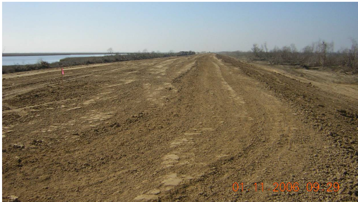
Figure 10.15: Levee rehabilitation work (location 4 on Figure 10.6) post Hurricane Katrina. The “semicompaction” construction approach was employed, utilizing earth moving equipment to also compact the placed material as it transported borrow materials to the construction site.
