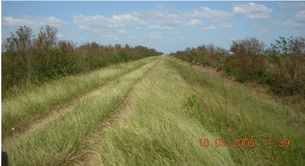
Figure 10.12: Condition of levees east of HWY 11 (location 3 on Figure 10.6) in October 2005. These levees performed exceptionally well and were not eroded during Hurricanes Katrina or Rita.
