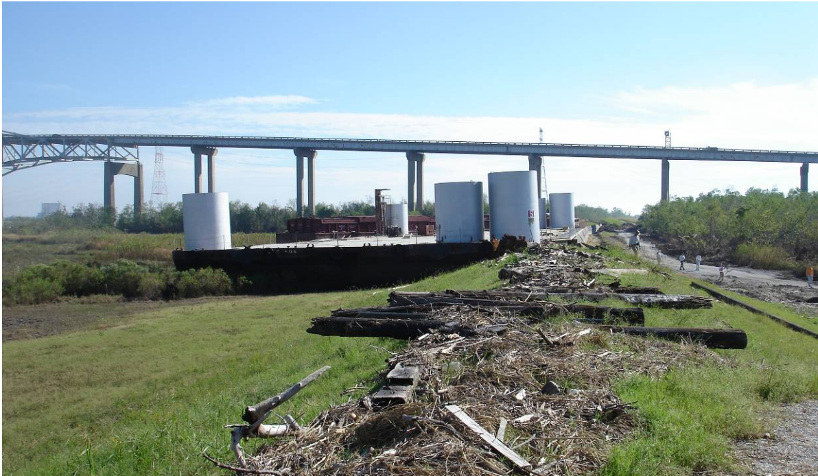
Figure 10.19: Woody debris and steel barges “washed up” on the southern ICWW/MRGO levee just west of Route 47 (location 6 on Figure 10.6). This is a side view from the aerial photograph presented in Figure 9.24.
