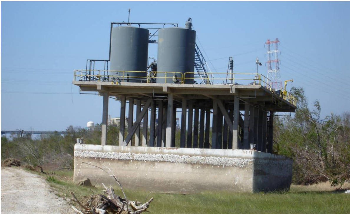
Figure 10.20: A gas processing barge “washed up” on the southern IWW/MRGO levee just east of Route 47 (location 6 on Figure 10.6). This levee was also overtopped and was not significantly damaged by the barge impact.
