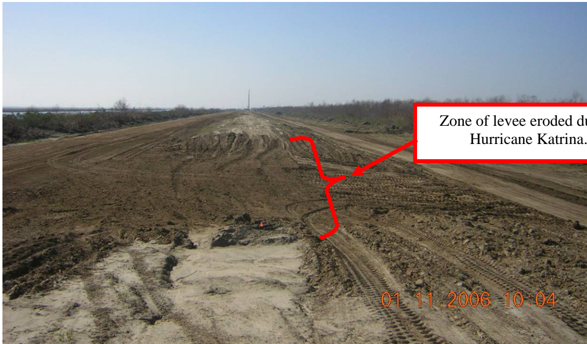
Figure 10.14: Zones of earthen levees at the southeast corner of the New Orleans East polder (location 4 on Figure 10.6) were washed out during Hurricane Katrina allowing water to rush in.
