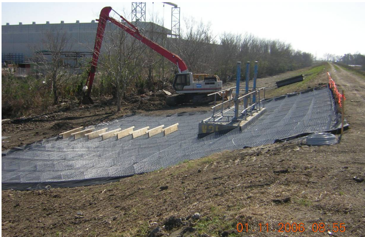
Figure 10.13: Levee rehabilitation work (near location 3 on Figure 10.6) after Hurricane Katrina included reinforcement and protection of soil-structure interactions with rock-gabion transition zones.
