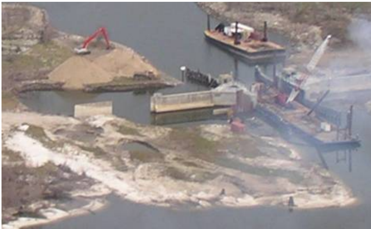
Figure 10.33: Close up aerial photograph showing backfilling operations at Bayou Dupre.
