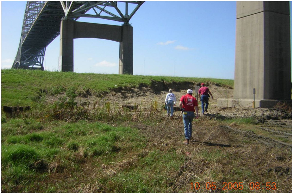
Figure 10.17: Post Hurricane Katrina view of the earthen levee shown in Figure 10.16. Only minor damage on the protected side was observed, with the majority of the damage a result of wave reflection from the bridge abutment at the right-hand side of the picture.
