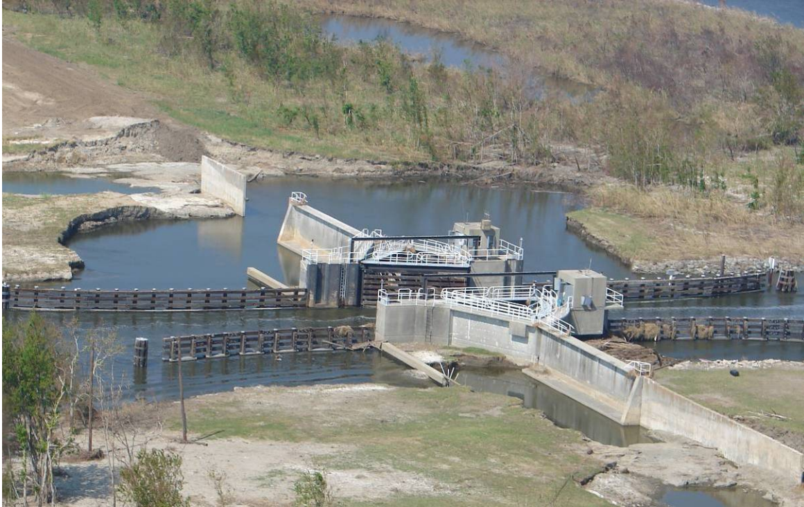
Figure 10.29: Control structure at Bayou Dupre (location 9 on Figure 10.6) suffered extensive scour and erosion during the storm surge and overtopping conditions associated with Hurricane Katrina.
