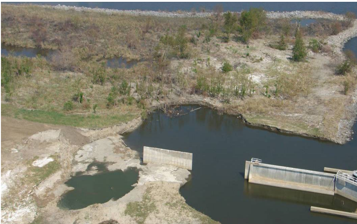
Figure 10.30: Another aerial photograph of the scour and erosion damage to the Bayou Dupre control structure.
