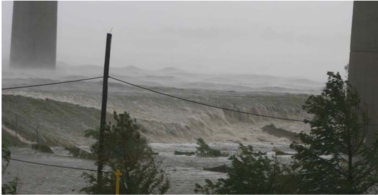
Figure 10.16: Photographs (location 5 on Figure 10.6) captured by a security camera at the Entergy Michoud Generating Plant beneath Route 47, on the IWW/MRGO show active overtopping during Hurricane Katrina.
