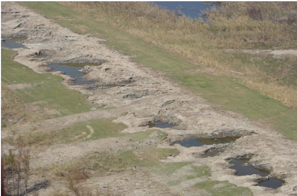
Figure 10.28: Close up aerial photograph of severely eroded MRGO levees at location 8 on Figure 10.6.
