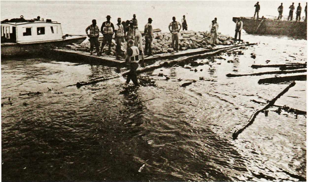
"Walking on the Water." Evenly distributed crushed rock gradually sinks a willow mat beneath the water. (Photo by C. Fortier)
