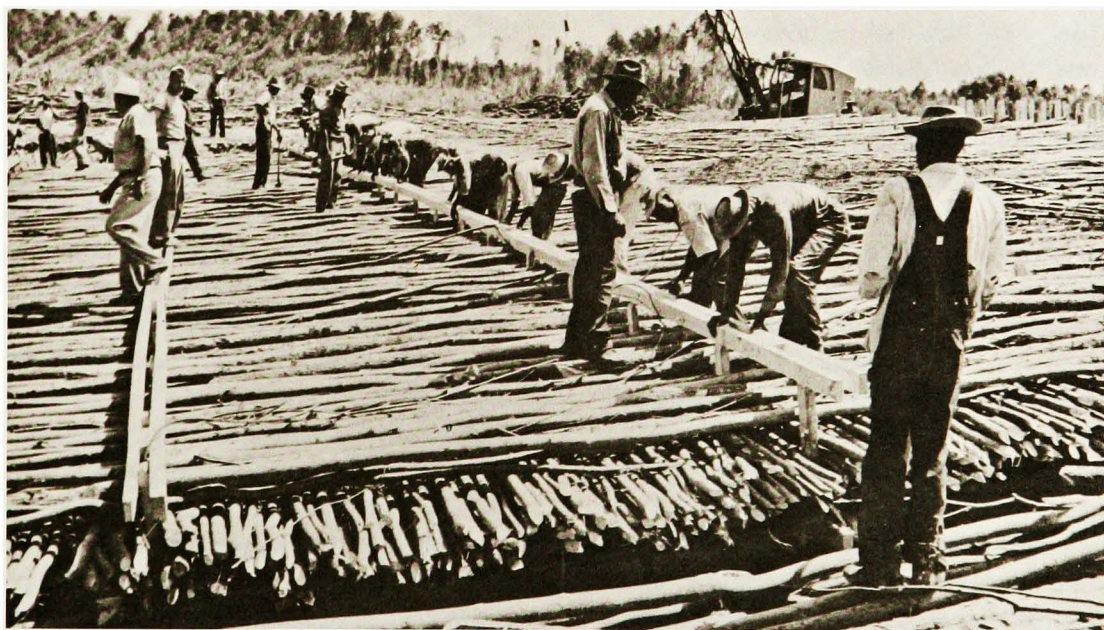
Bank protection—old style. Weaving of a giant willow mattress.
