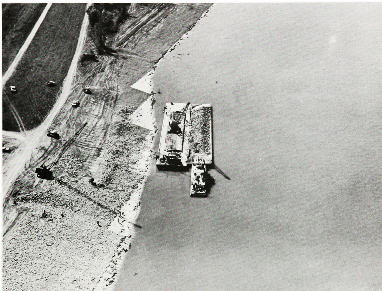
Bank protection—new style. Riprap (broken stone) is laid to overlap the articulated concrete mats.
