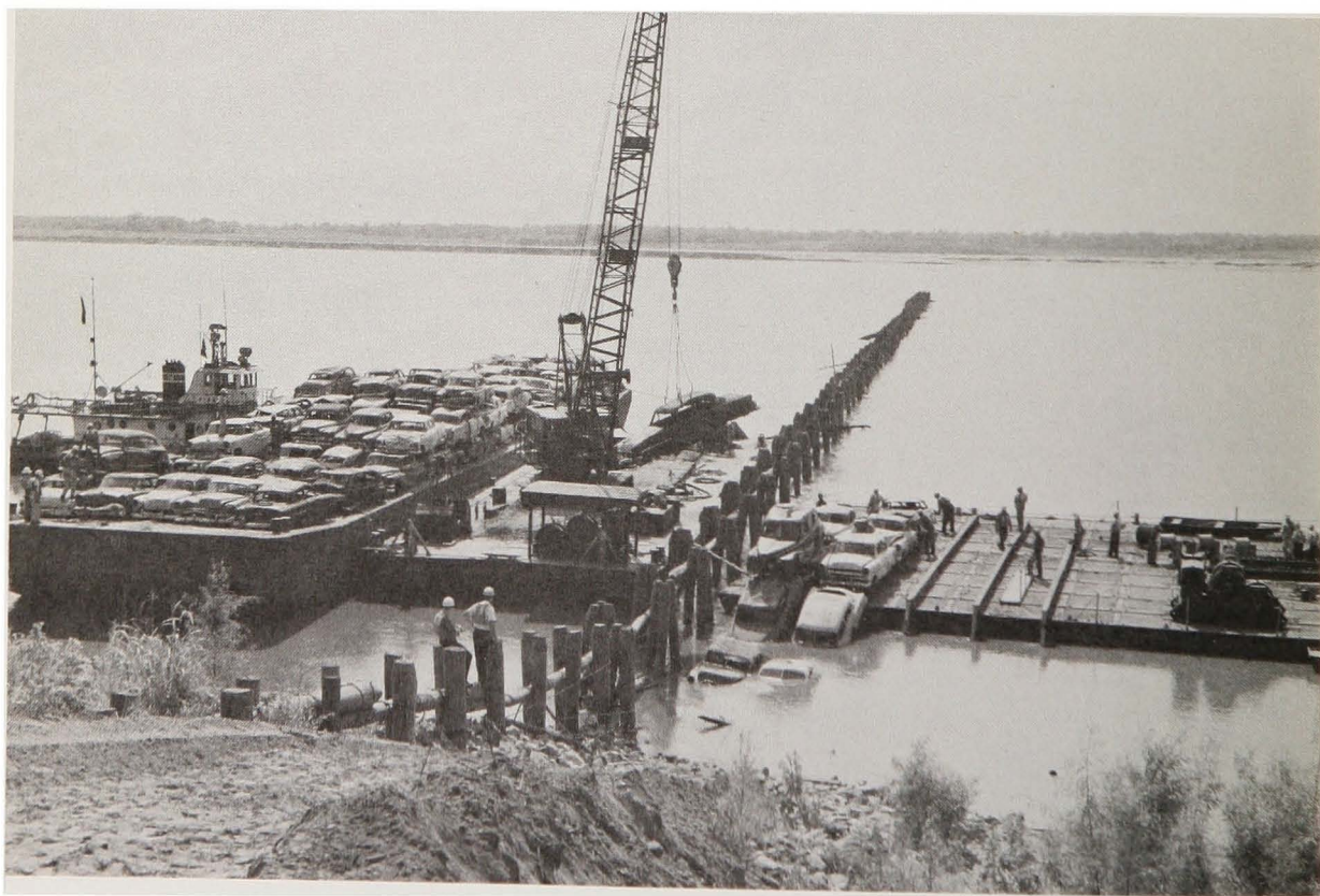
Figure 66. Car body dike placement along upstream side of existing dike
