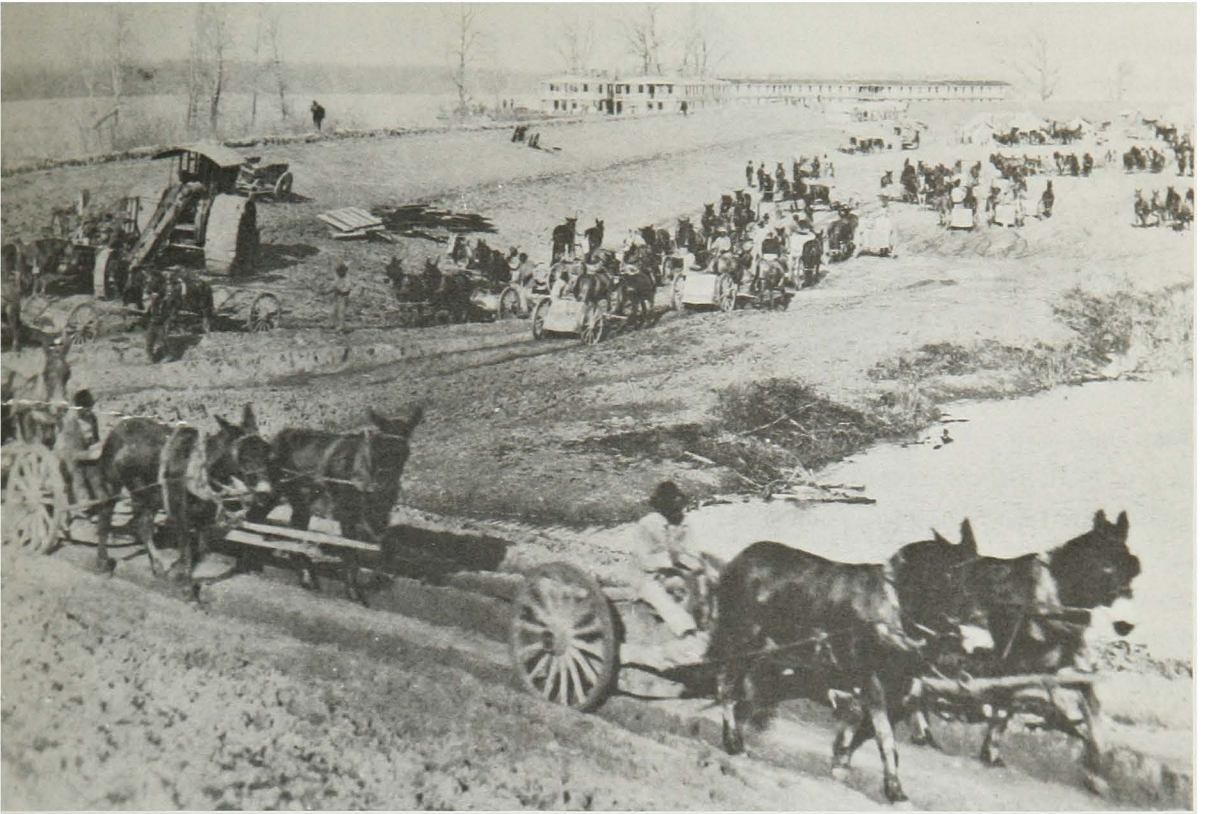
Figure 45. Manpower—and mulepower—required for construction of early levees in lower Mississippi River Valley
