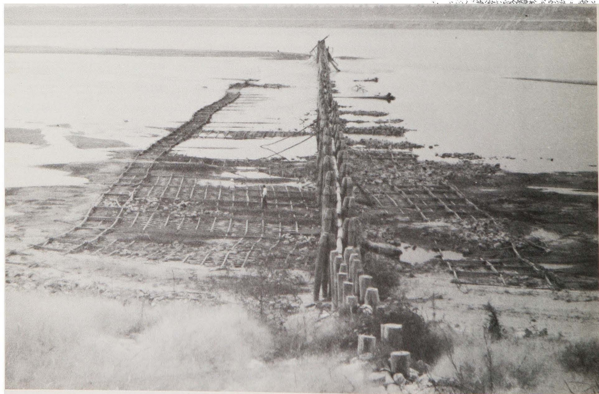
Figure 64. Foundation mattress for pile dike construction
