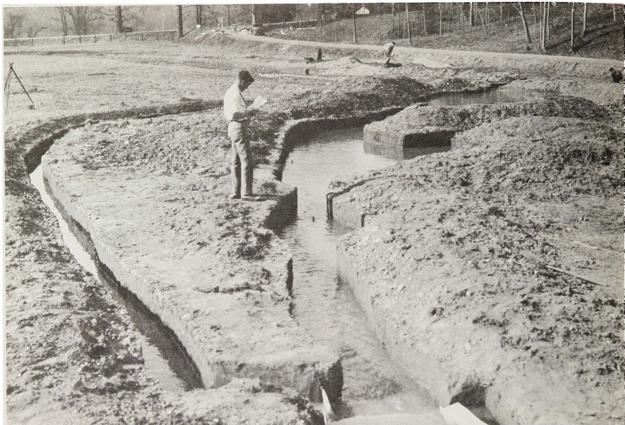
Figure 37. First model at the Waterways Experiment Station: Determination of Mississippi River backwater limits on Illinois River above Grafton, Illinois
