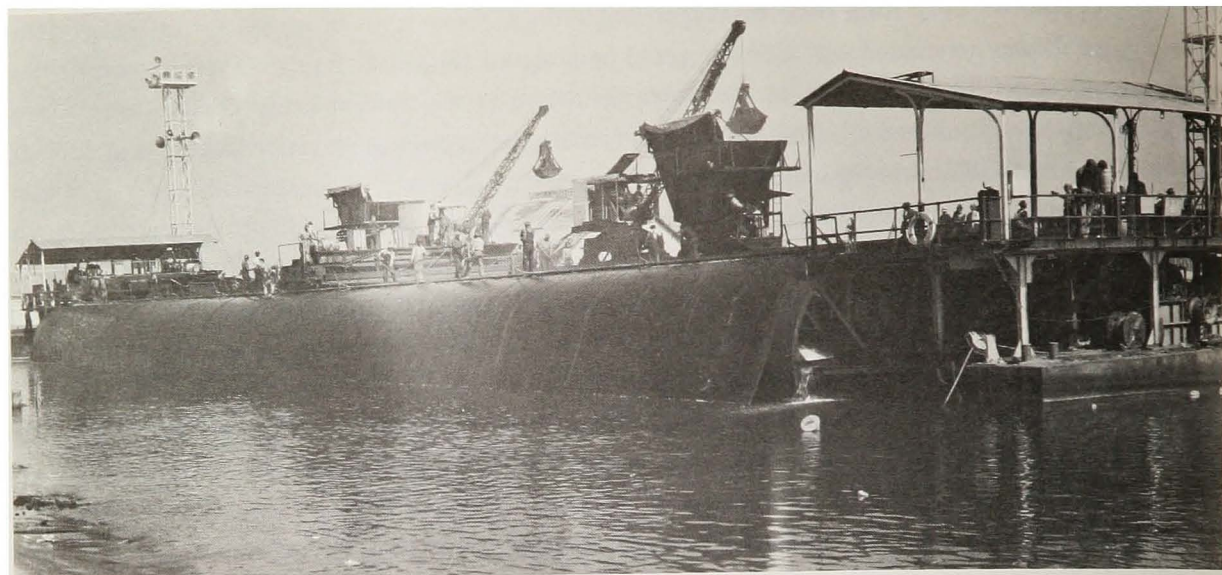
Figure 16. Launching reinforced asphalt mattress
