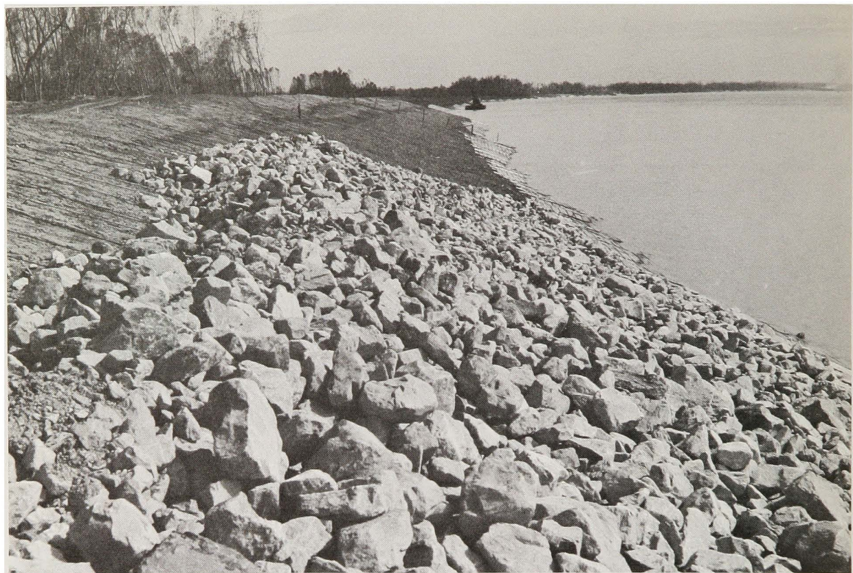
Figure 61. Riprap upper bank paving
