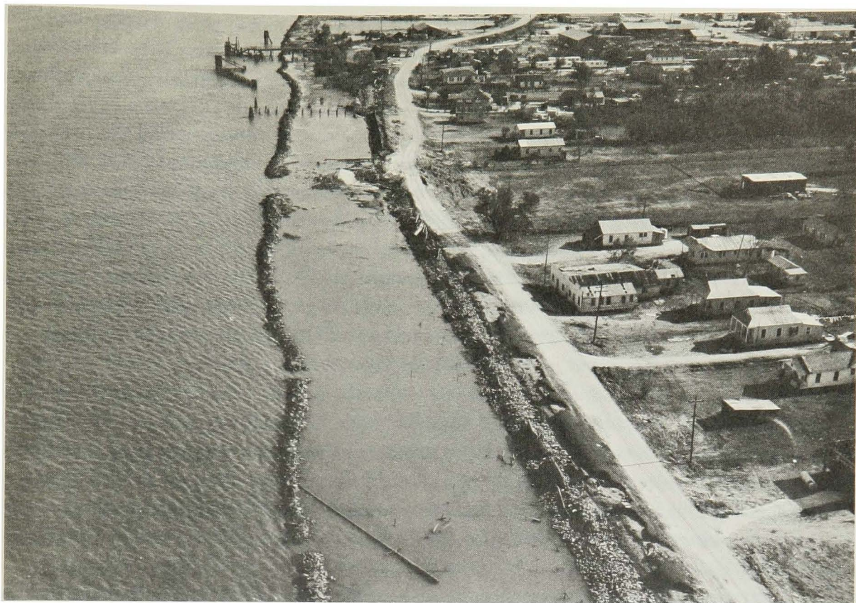
Figure 74. Typical scene of damage to levees on lower Mississippi River by Hurricane Betsy
