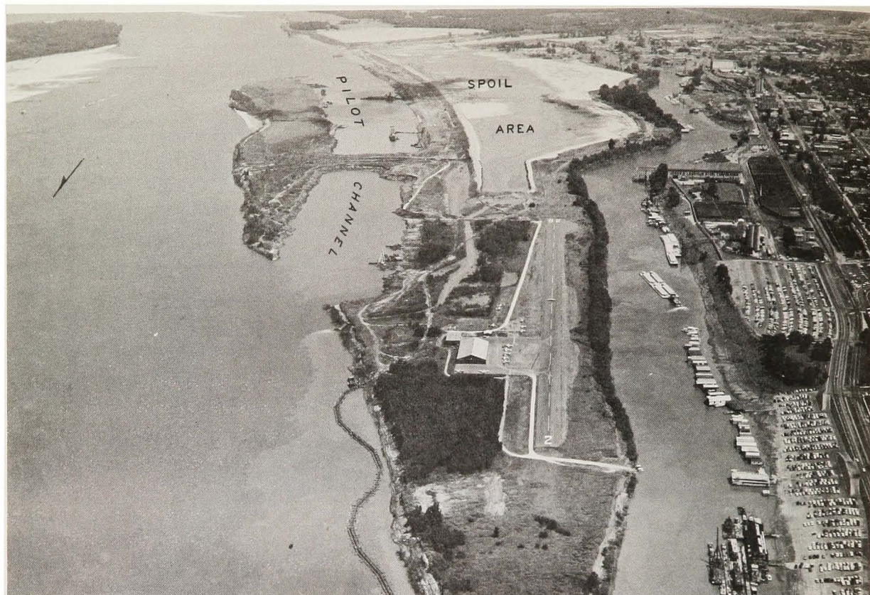
Figure 70. Dredging pilot cut for new navigation channel, Memphis
