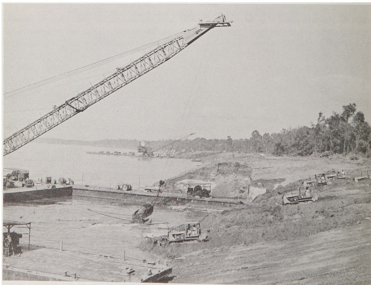
Figure 57. Bank grading in preparation for placement of revetment
