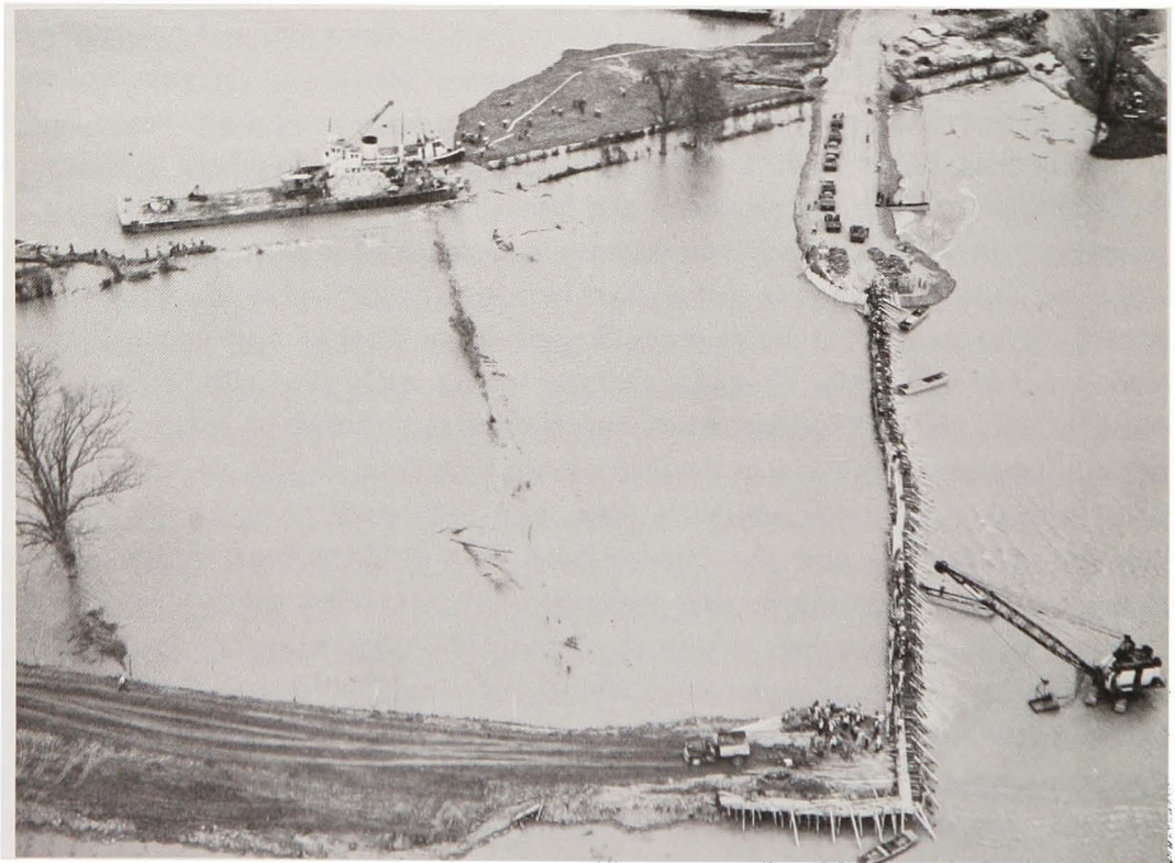
Figure 31. Temporary closure of Free Nigger Point crevasse
