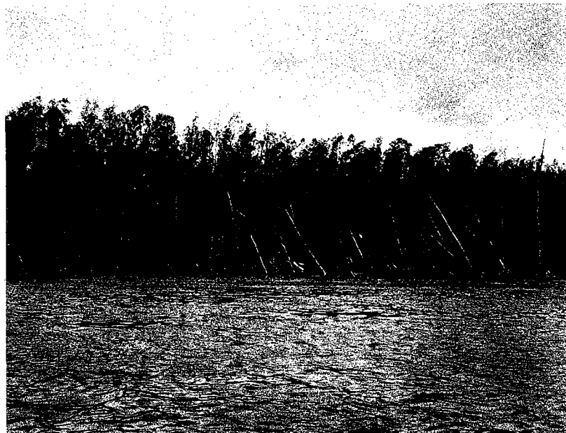
Fig. 24. Slumping of backswamp materials at river mile 66. The slump block has subsided beneath the water, but the trees which grew upon it and the angle which they make with the vertical indicate its extent and the relative position. Photograph taken 1 December 1950
