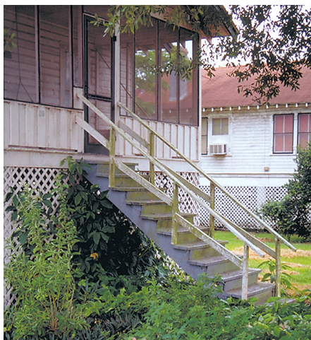
Figure 7. This building at the Everglades Experiment Station was originally constructed at the land surface; latticework and stairs were added after substantial land subsidence.
