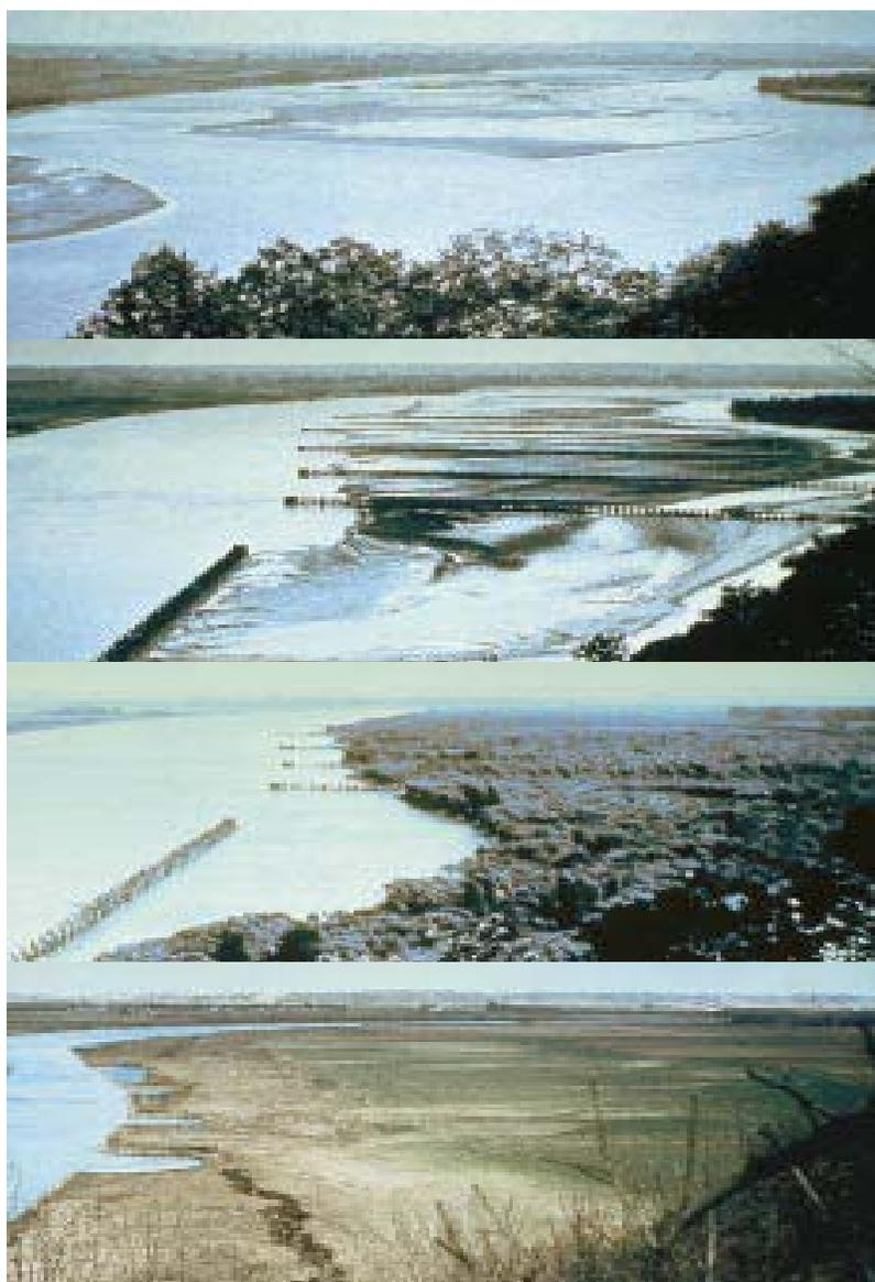
FIGURE 2-5 Photographs taken at Indian Cave Bend on the Missouri River near river mile 517, about 18 miles upstream from Rulo, Nebraska. They illustrate the river before (1934; top photo) and after (1935, 1946, and 1977) the construction of brush dikes that narrowed and channelized the river. View is looking downstream from Nebraska (near bank) into Missouri (far bank). These photos illustrate substantial alteration of riparian and in-channel habitats. SOURCE: USGS, 1998.
