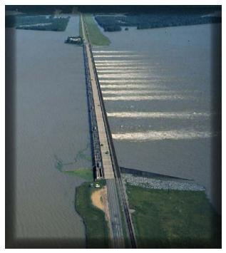
remain operable at all river stages, but the overbank structure is only operated during flood stages. During project flood conditions, the Old River Control Complex is designed to divert 620,000 cfs from the Mississippi River to the Atchafalaya River.
