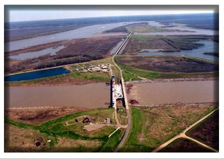
project flood peak stages. When flood stages on the Mississippi River or its tributaries subside, floodwaters from within the backwater areas evacuated through floodgates.
