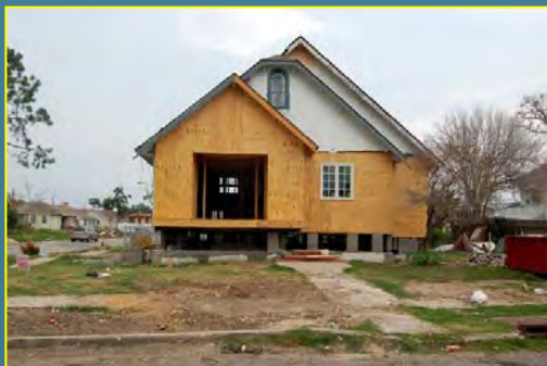
Protect Substantially Damaged
