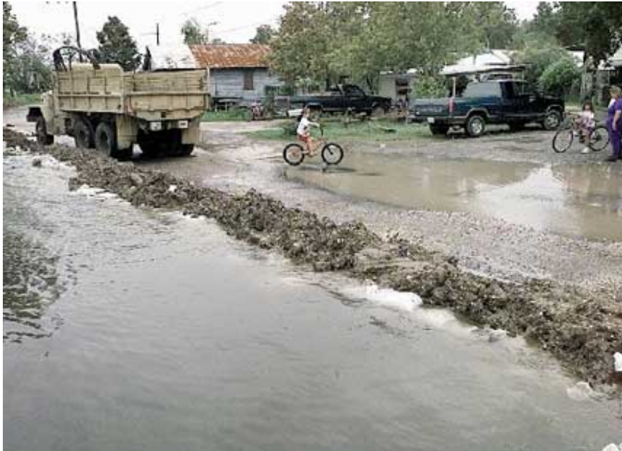
Keeping roads passable and homes dry is a constant battle for state, local and federal officials. Here, St. Charles Parish officials and the National Guard hastily constructed a 2-foot levee to keep floodwaters from Tropical Storm Frances away from homes on Up the Bayou Road in Des Allemands in September 1998. (PHOTO BY THOM SCOTT / The Times-Picayune)
