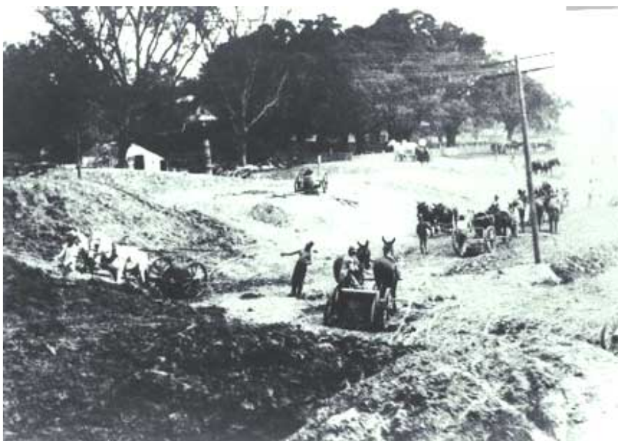
LEVEE-BUILDING IN 1908 - workers using mules and horses haul dirt to raise a levee in Jefferson Parish in 1908. The next year, an unnamed storm killed 353 people when a 15-foot storm surge inundated much of South Louisiana.
