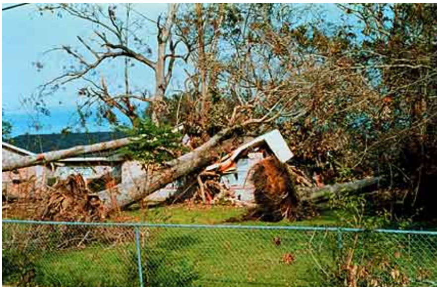
Trees downed by Hurricane Andrew destroyed these homes north of Avery Island in Louisiana. Fortunately the residents had fled. (NWS ARCHIVE PHOTO)
