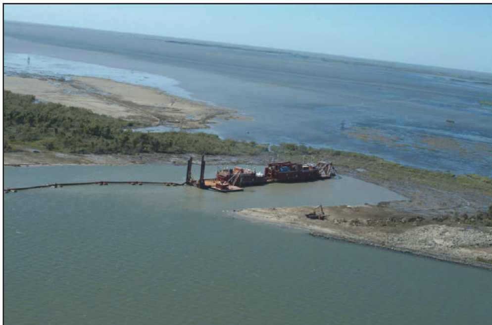
Figure 1.3. WBSD channel under construction.
