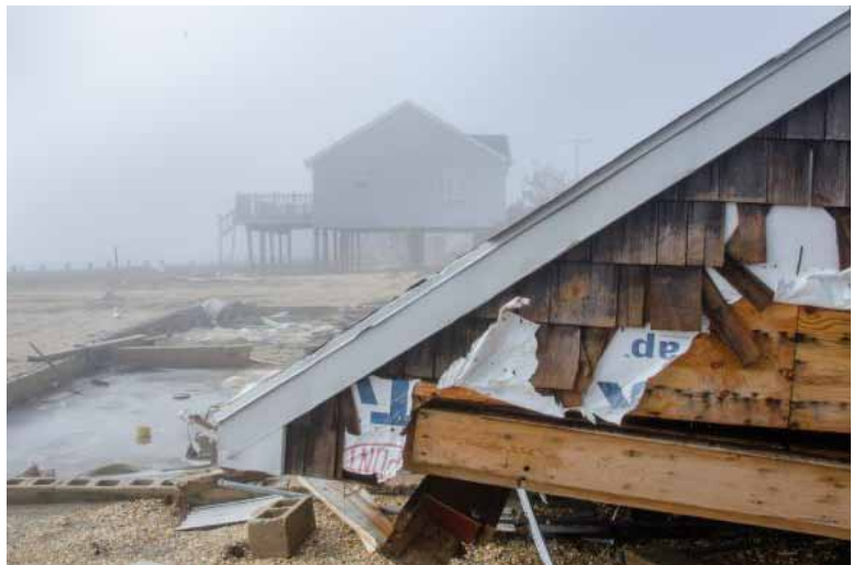
Ocean Gate, N.J., Jan. 30, 2013 -- The home on pilings, in the background, survived Hurricane Sandy with relatively little damage, while its neighbor (foreground) was not as fortunate. Photo by Liz Roll/FEMA
