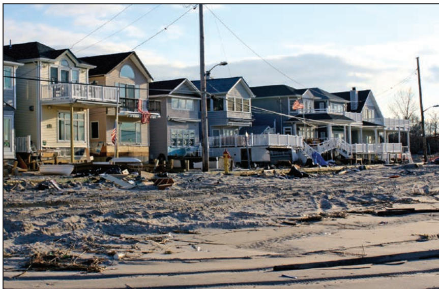
Figure 1: Homes on small, tightly spaced lots, typical throughout coastal New York and New Jersey, present access and construction challenges when being transitioned to a raised pile foundation (Rockaway, NY)
