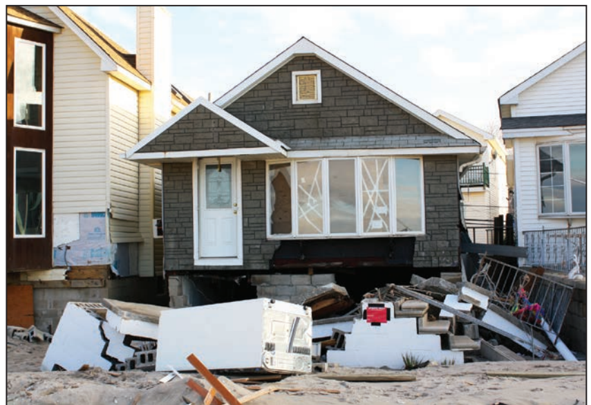
Figure 5: Elevating tightly spaced homes, such as these in Breezy Point, NY, presents construction challenges
