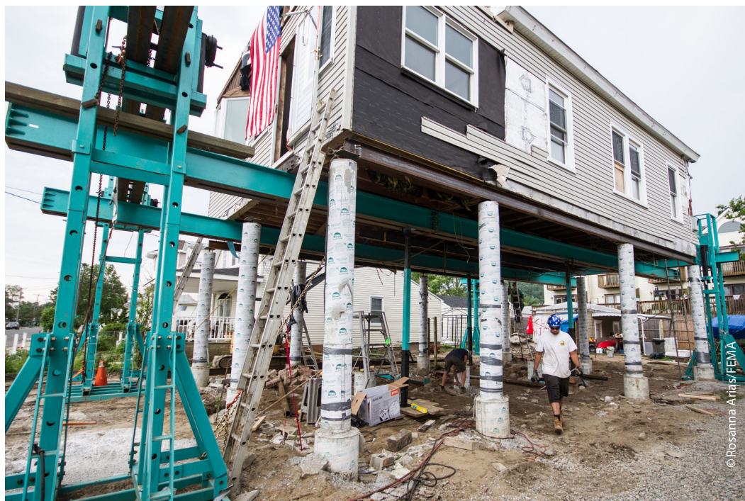
Some New Jersey home owners are opting to elevate their homes in the wake of Hurricane Sandy and the implementation of the Biggert-Waters Flood Insurance Reform Act of 2012 (see box above). Elevation not only better protects homes from storm surge and subsequent flooding, but can also help reduce insurance premiums for home owners.
