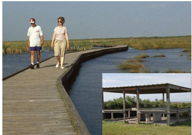
This marsh boardwalk and fish cleaning station are similar to structures in the Sea Rim State Park Improvements project in Texas.
