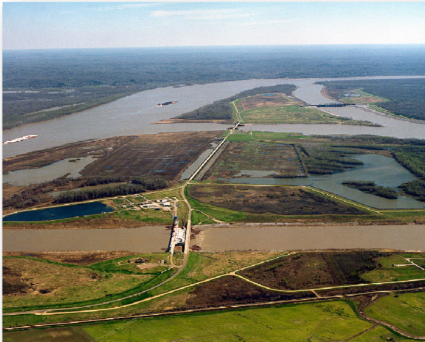
Old River Control Structure
