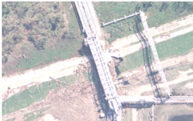
Figure 10. Mississippi River Levee Breach at ConocoPhillips Refinery during Katrina
