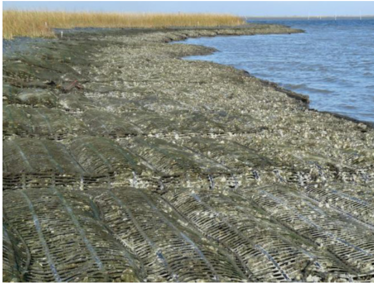
Figure 5.D-9. Gabion mats with oyster shell used to restore fringing oyster reefs for the North Shore of Terrebonne Bay, Louisiana.
