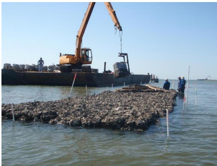
Figure 5.D-11. Crews deploying oyster reefs along Coffee Island in Portersville Bay near Bayou LaBatre, Alabama.
