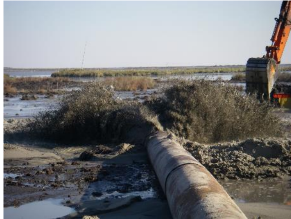
Figure 5.D-2. Dredged sediment pumped via pipeline to the CWPPRA Bayou Dupont restoration project, Mississippi River Sediment Delivery System—Bayou Dupont (BA-39), Jefferson and Plaquemines Parishes, Louisiana.
