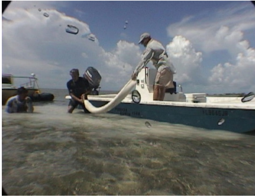
Figure 5.D-13. Restoration team deploying biodegradable sediment filled tubes to restore sediment grade and seagrasses in a vessel grounding site.
