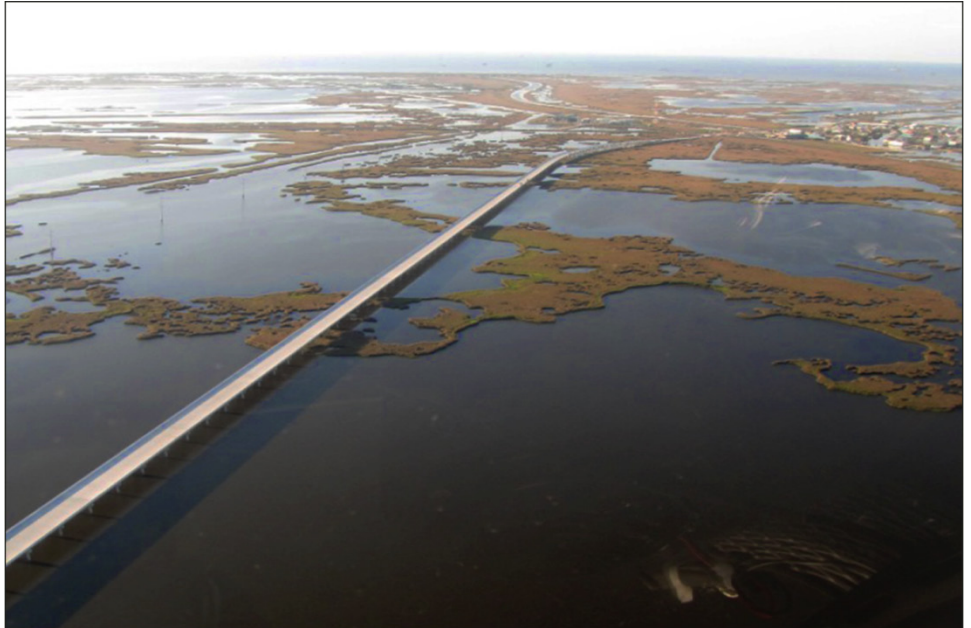
Figure 3: Louisiana State Highway 1 Leading to Port Fourchon
