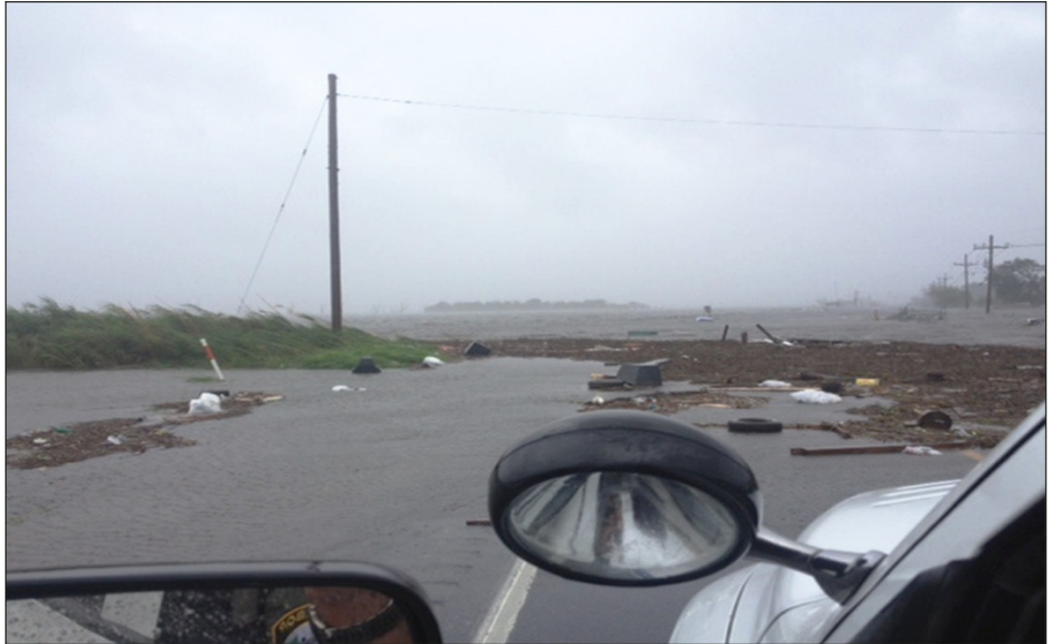
Figure 11: Flooding of an Unraised Segment of Louisiana State Highway 1 Following Hurricane Isaac
