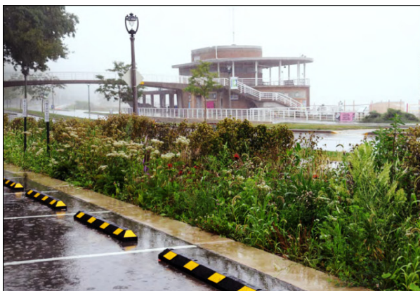
Bio-swale – a depressed catchment area planted with vegetation that captures and infiltrates runoff.
