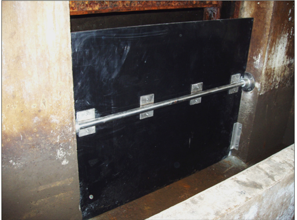
Figure 13: Flap Gate Installed at the Barton Pump Station
