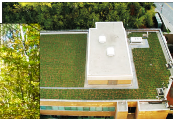
Green roof – a roof either partially or completely planted with vegetation growing in soil (or a growing medium) to hold rainwater.
