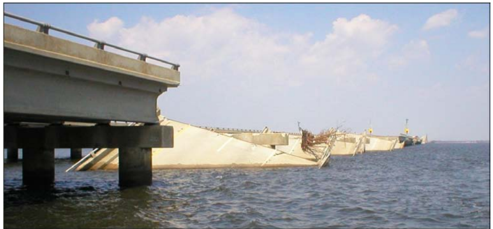
Figure 1: Damaged Segments of the Twin Span Bridge
