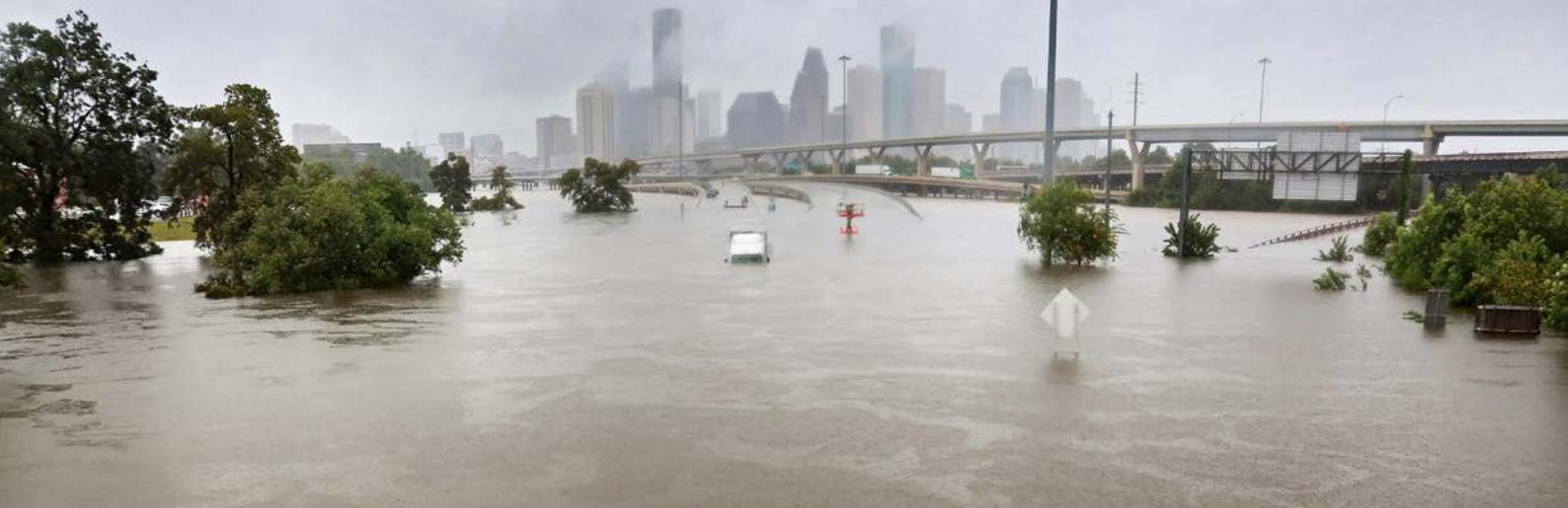
Freeways in Houston submerged under water following Hurricane Harvey
