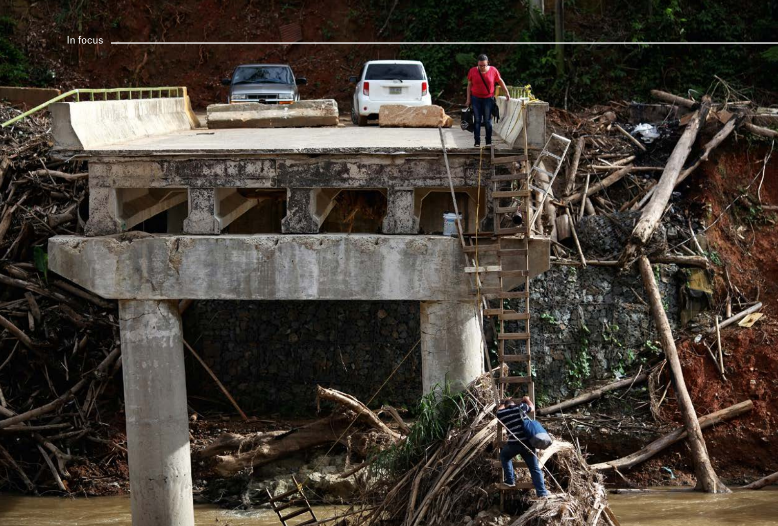
Bridge in Puerto Rico after Hurricane Maria hit the area in September 2017
