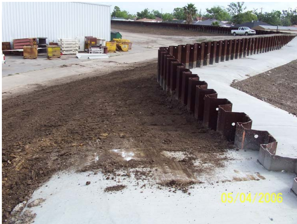
Figure 25-6 – Overtopping Scour Protection for Sheetpile I-wall
