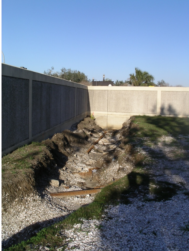
Figure 25-5 – Overtopped Type II I-Wall with Damage but No Failure
