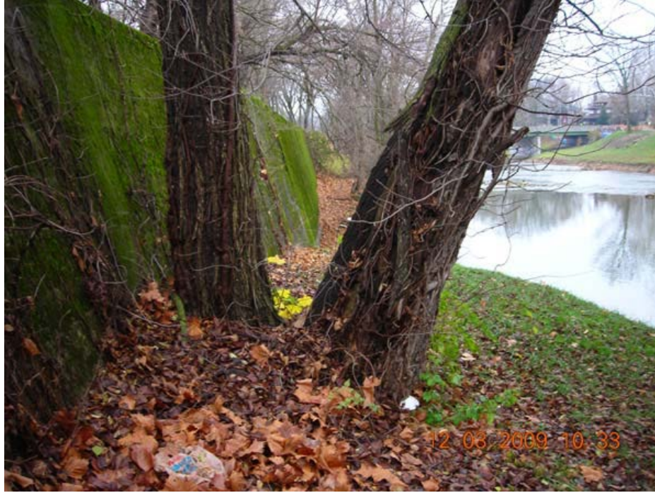
Figure 25-7 – Large Trees Adjacent to Floodwall
