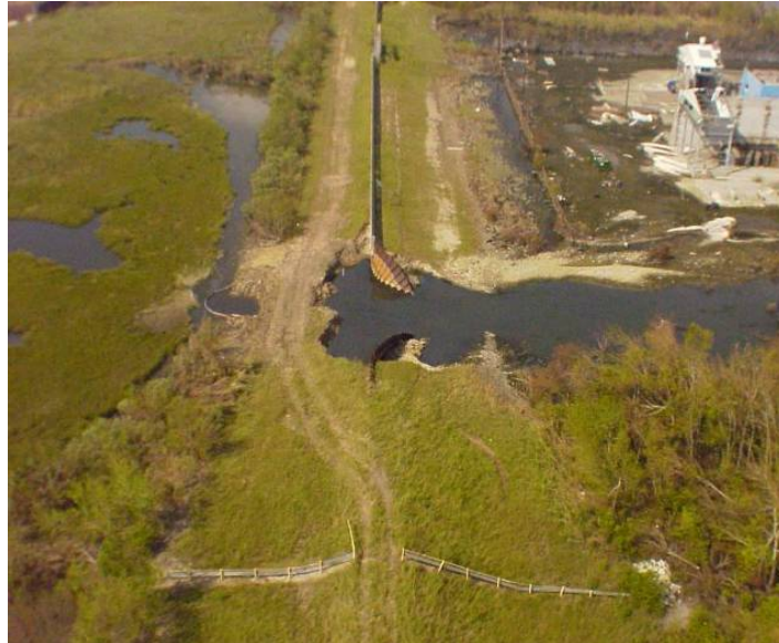
Figure 25-4 - Failure of Sheetpile I-wall due to Overtopping
