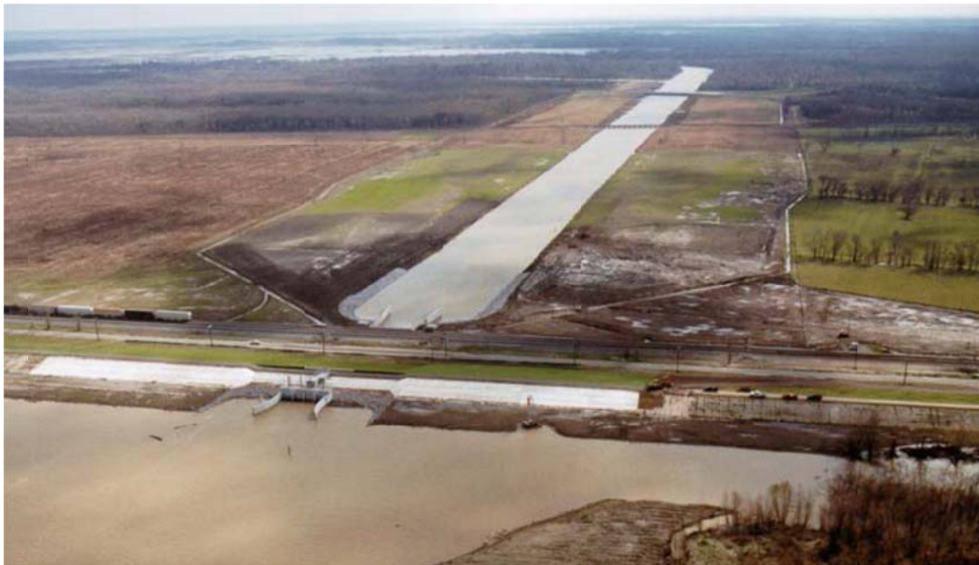
Figure 1-3. Photo of Davis Pond (capable of diverting up to 8,800 cfs) (from LDNR 2003)
