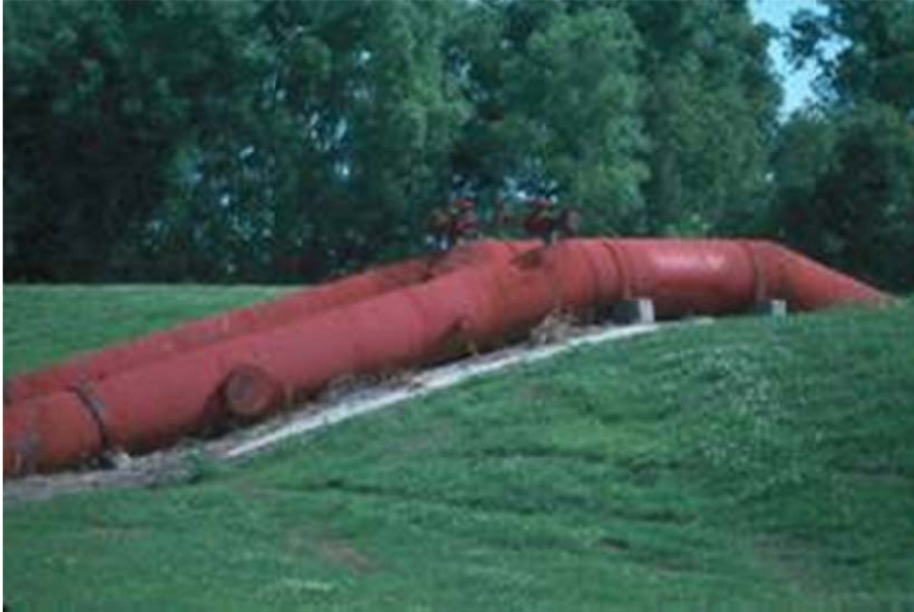
Figure 1-10. Photo of White's Ditch Siphon (capacity 200 cfs) (from Center for Environmental Communications, Loyola University 2010)
