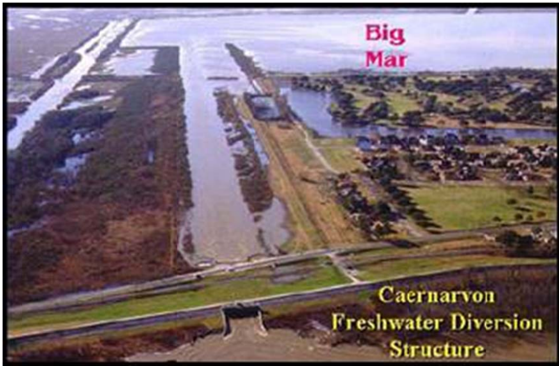
Figure 1-2. Photo of Caernarvon (capable of diverting up to 10,650 cfs) (from CPRA 2010)
