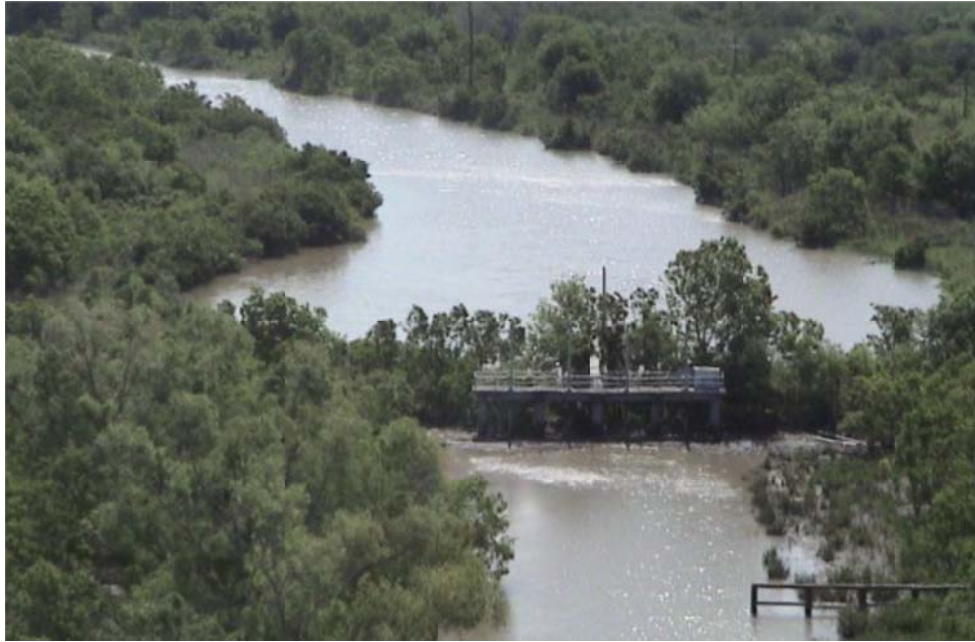
Figure 1-4. Photo of Bayou Lamoque Diversion (capacity 12,000 cfs). Currently in disrepair, unauthorized operation except for oil spill. (from Louisiana Coastal Wetlands Conservation and Restoration Task Force 2007)
