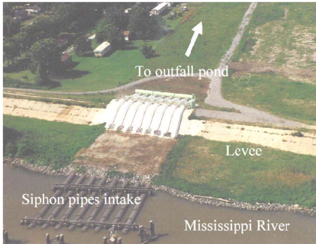
Figure 1-12. Photo of West Pointe a la Hache Siphon (capacity 1,500 cfs) (from C.H. Fenstermaker & Associates, Inc. 2004)
