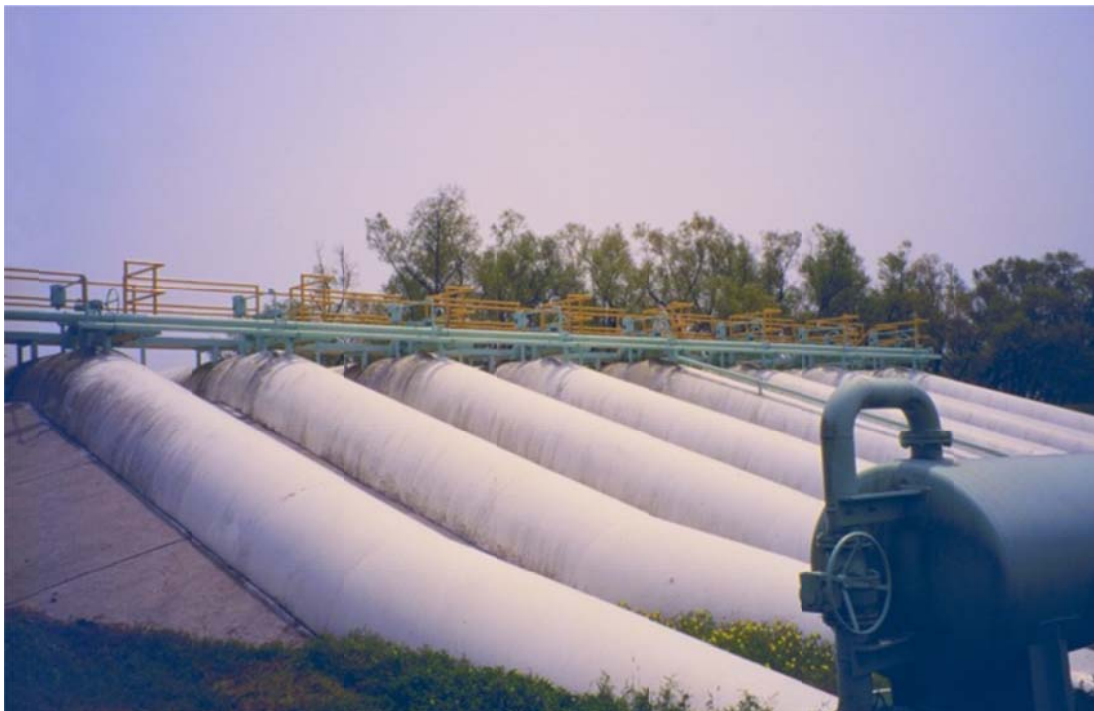
Figure 1-11. Photo of Naomi Siphon (capacity 1,500 cfs) (Source: NOAA 2010)
