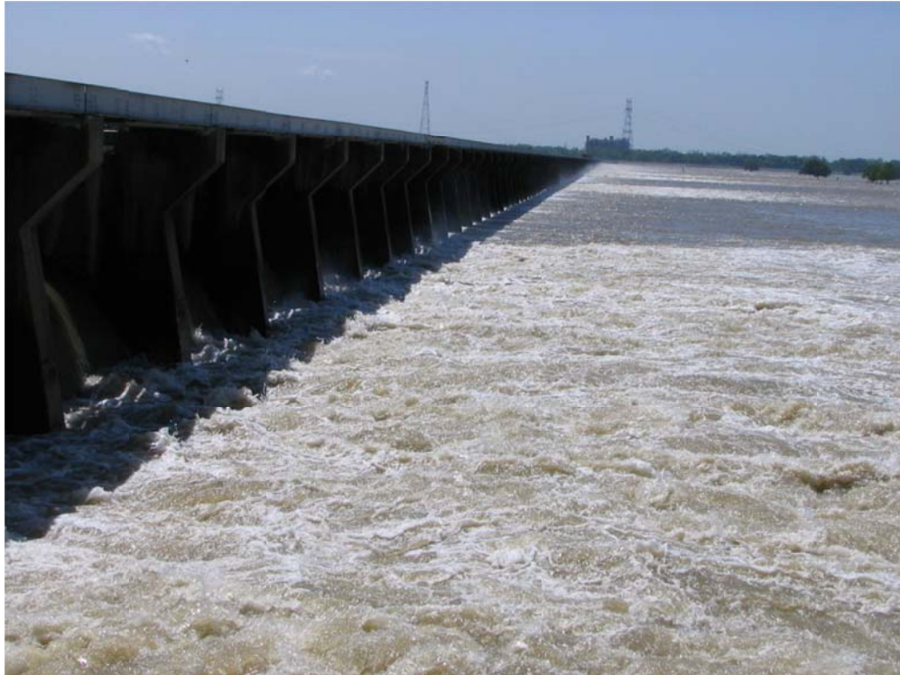
Figure 1-13. Bonnet Carré Spillway during 2008 Opening (design capacity 250,000 cfs) (Source: G.E.C. Inc.)
