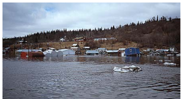
Flooding in Russian Mission. Photograph courtesy M. Bird, ADES.
