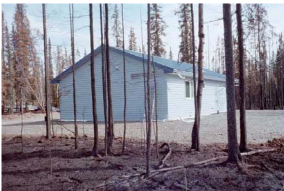
Tok, AK. Defensible space surrounding this house helping make it FireWise. Image courtesy of Alaska Visitor Information Services.
