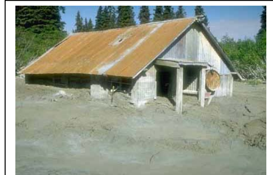
Lahars from the 1989 to 1990 eruptions of Redoubt Volcano inundated this structure near the mouth of Drift River. Photograph courtesy of C. Gardner, USGS.
