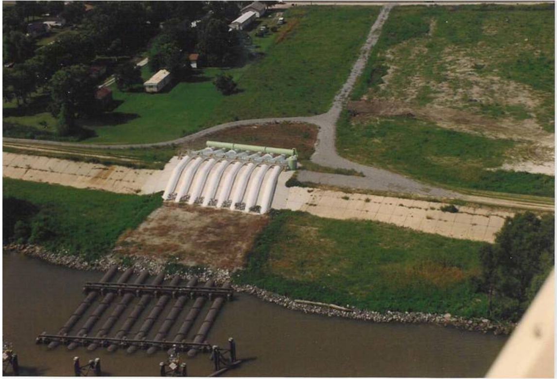
Figure 1. West Pointe a la Hache siphons (BA-04) constructed in 1992 and funded by the state of Louisiana. Mississippi River water was siphoned from the river intakes, discharged into a ponding area and distributed through 4 channels into the surrounding marshes.
