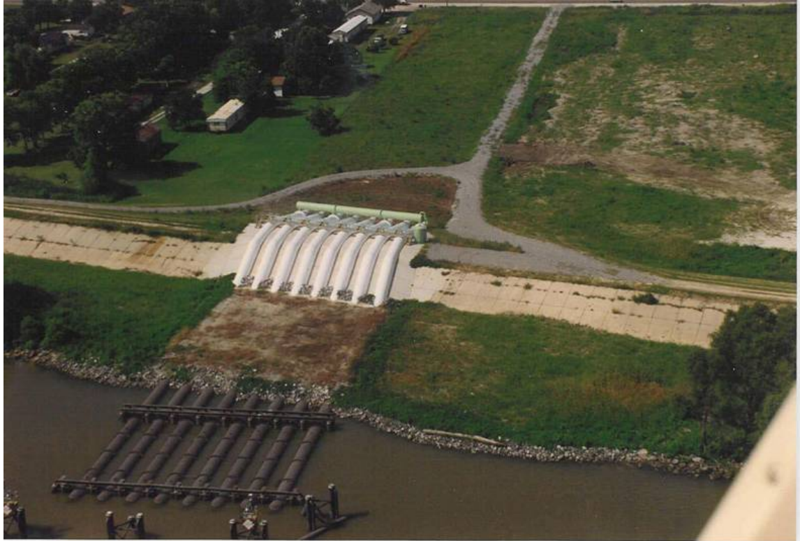
Figure 1. West Pointe a la Hache siphons (BA-04) constructed in 1992 and funded by the state of Louisiana. Mississippi River water was siphoned from the river intakes, discharged into a ponding area, and distributed through four channels into the surrounding marshes.
