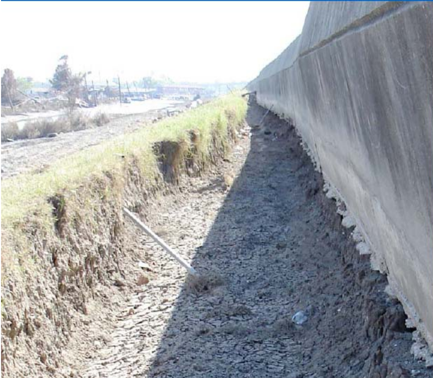
Figure 24. Example of breach along IHNC (east side) from overtopping and scour (top) and scour behind adjacent section that did not fail (bottom).
