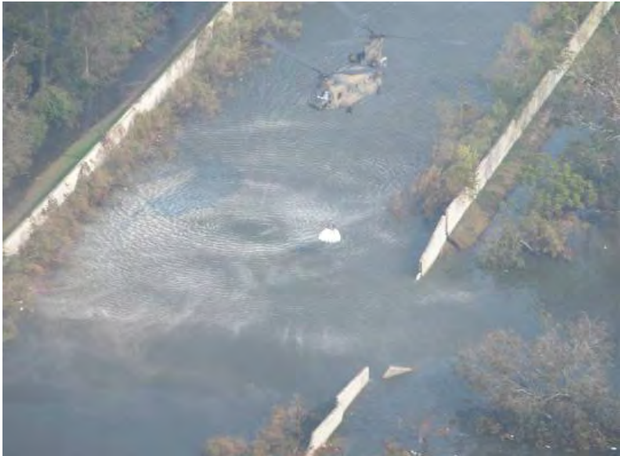
Figure 28. South Breach, London Avenue Canal
