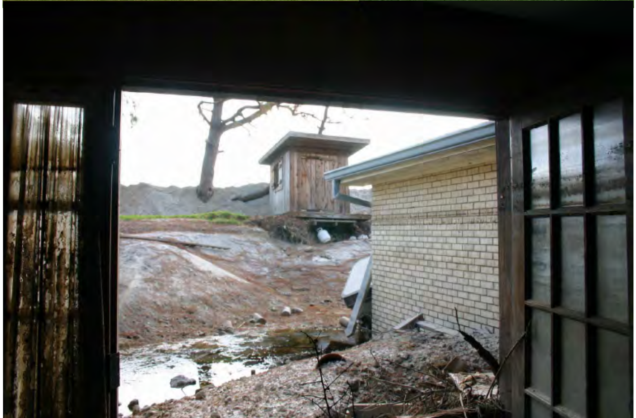
Figure 30. Playhouse at the London Avenue Canal North Breach Before the Failure (top photo) and After (bottom photo)
