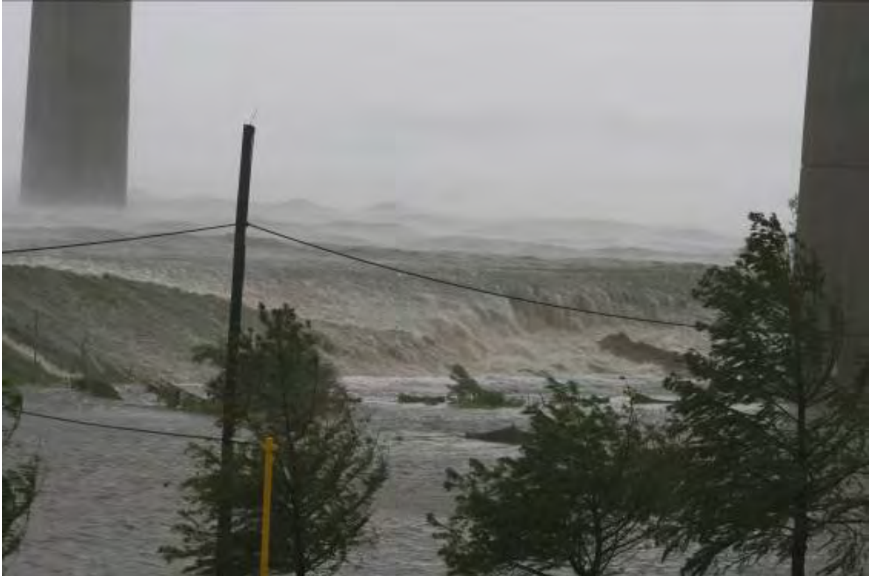
Figure 62. Overtopping of the Levee Under the Paris Road Bridge Adjacent to the Entergy Power Plant in the New Orleans East During Hurricane Katrina
