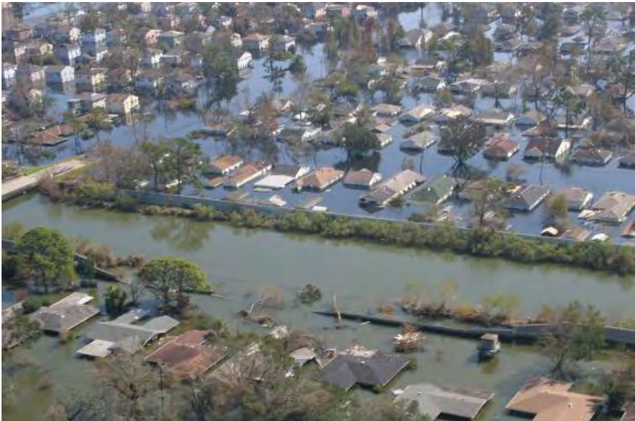
Figure 29. North Breach, London Avenue Canal
