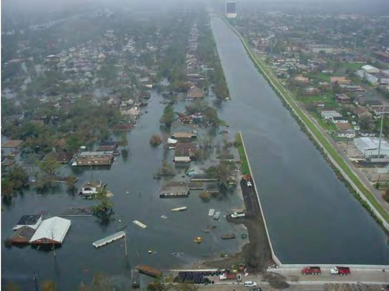
Figure 3. Aerial Photograph of the 17th Street Canal Breach Looking South From the Old Hammond Road Bridge
