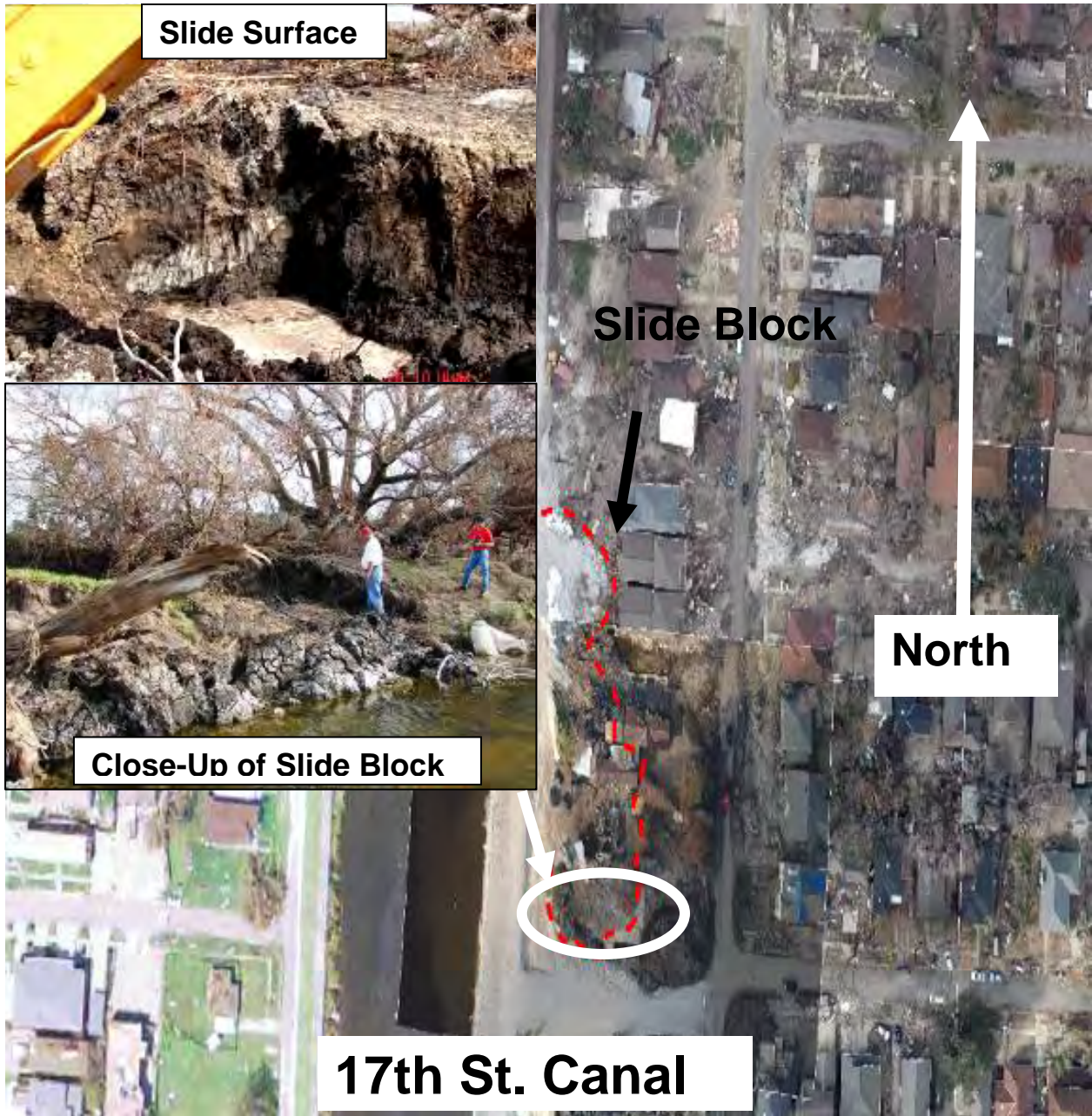
Figure 10. Photographs Taken at the 17th Street Canal Breach After the Failure
