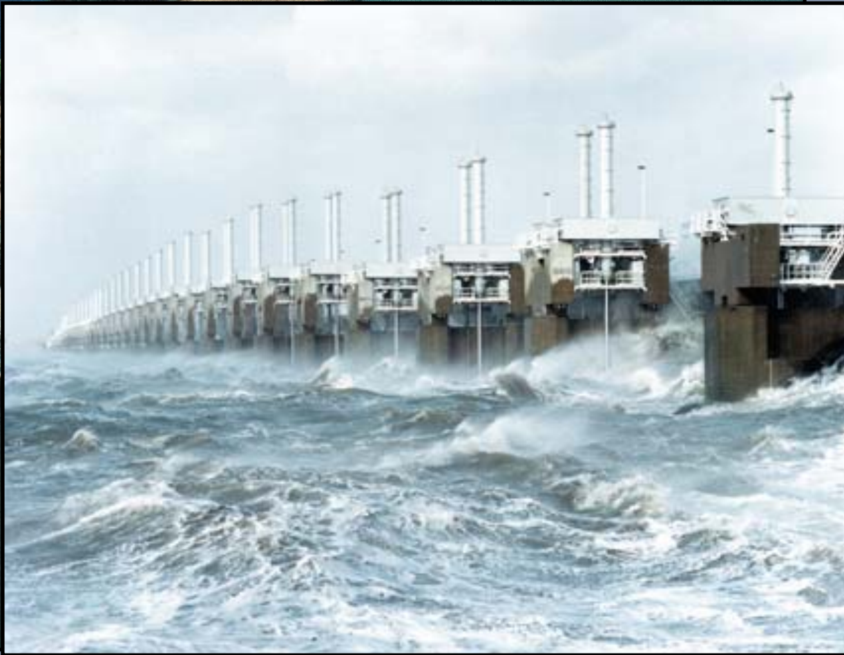
Easter Scheldt storm surge barrier 1986
