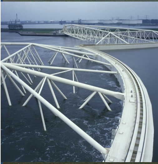
Maeslantbarrier; Accessibility Rotterdam harbor
