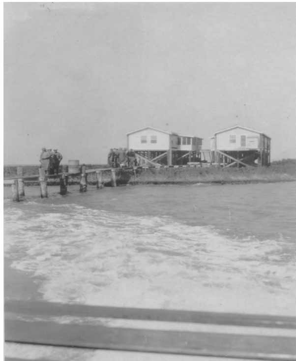
Figure 6. Field Office and Crew Quarters.
