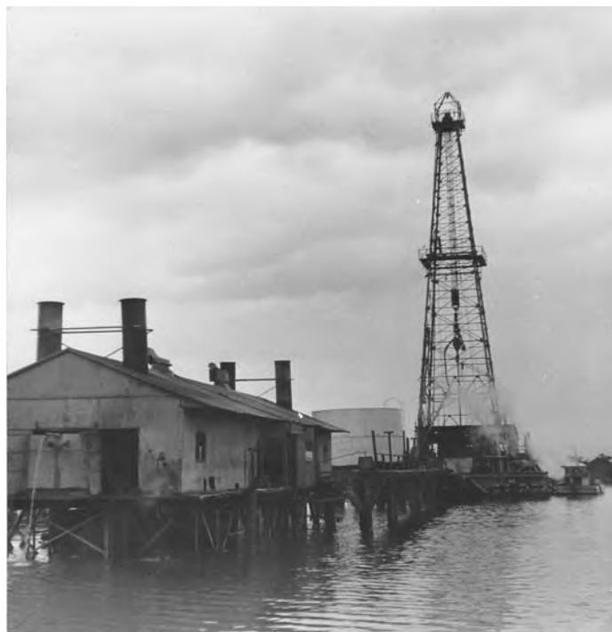
Figure 10. Barge Drilling Rig by Field Facilities.
