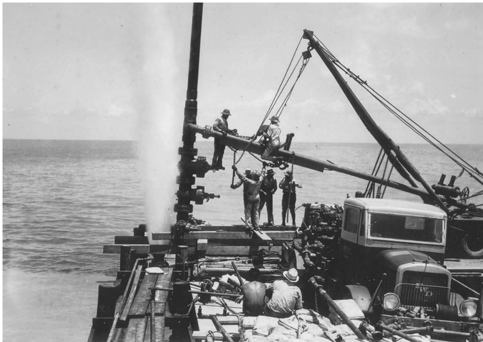
Figure 4. Working on a Blowout.
