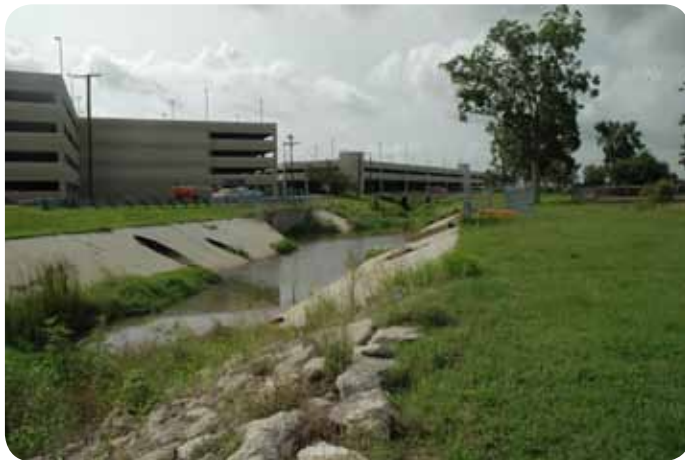
Figure 7: Bayou Monte Sano, Baton Rouge - Before and After Restoration
